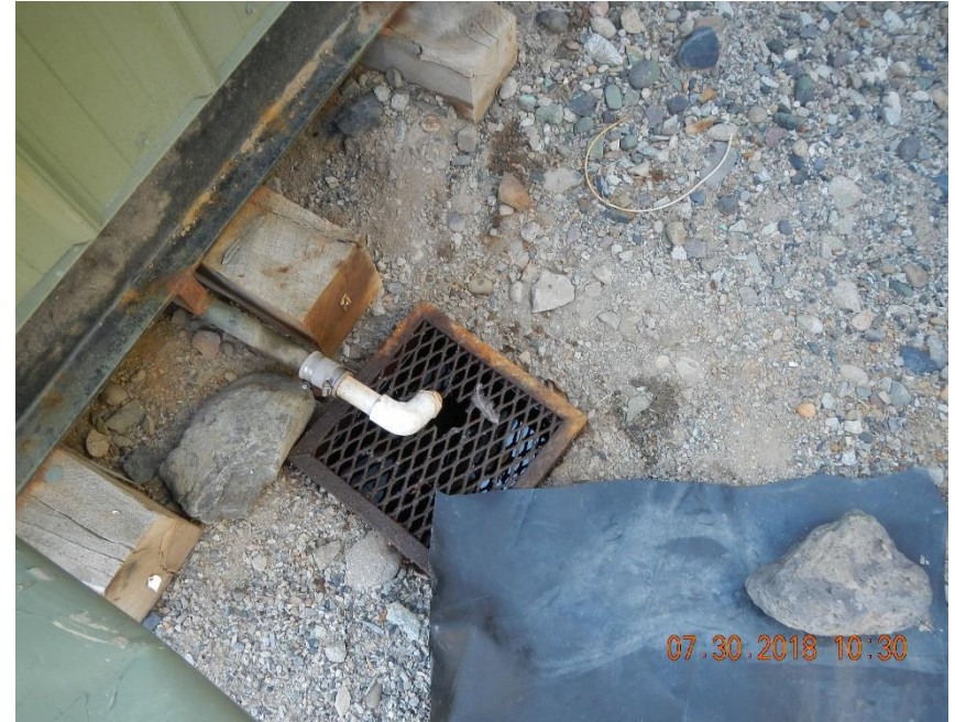
Equipment drain from transfer pump shack.
