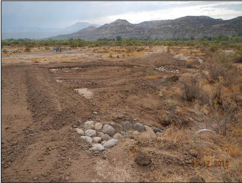
Photo 1. Stormwater controls installed on edge of location.
