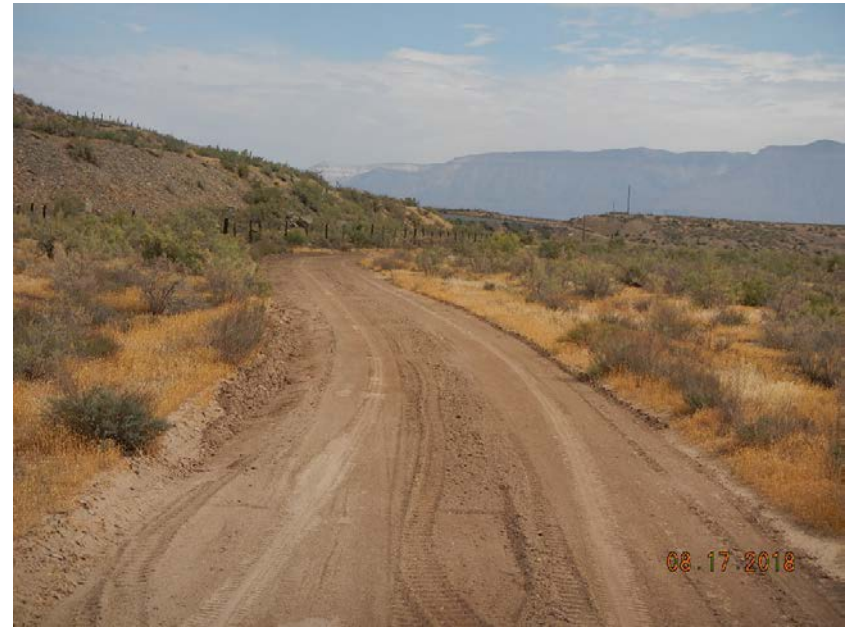
Photo 2. Road graded and bar ditch cleaned.
