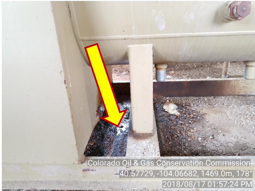
Photo #16 April 12-14 & Dryer 1 Soil stain appears below separator
