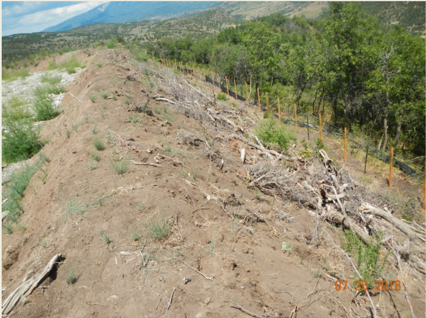
Photo 5. View of the eastern portion of the project area from the southeastern corner facing northward. Silt fence along the perimeter is in disrepair.
