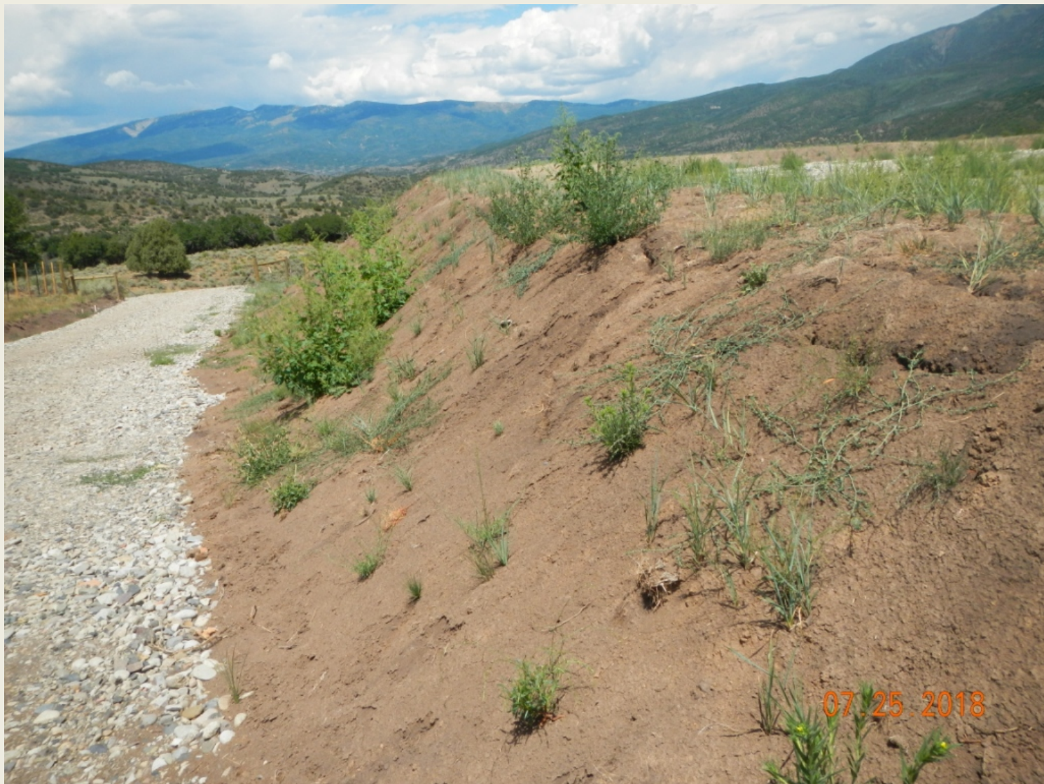
Photo 3. View of exposed soils at the northwester access entrance. This area needs better stabilization and sediment controls.
