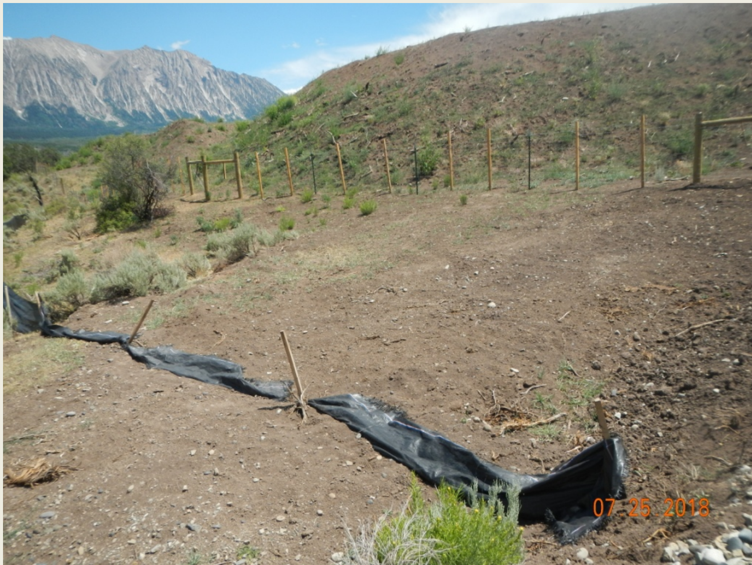
Photo 4. View of damaged silt fence and exposed soils that are not protected (also downslope from silt fence in lower left portion of photo), in the northwestern portion of the project area.
