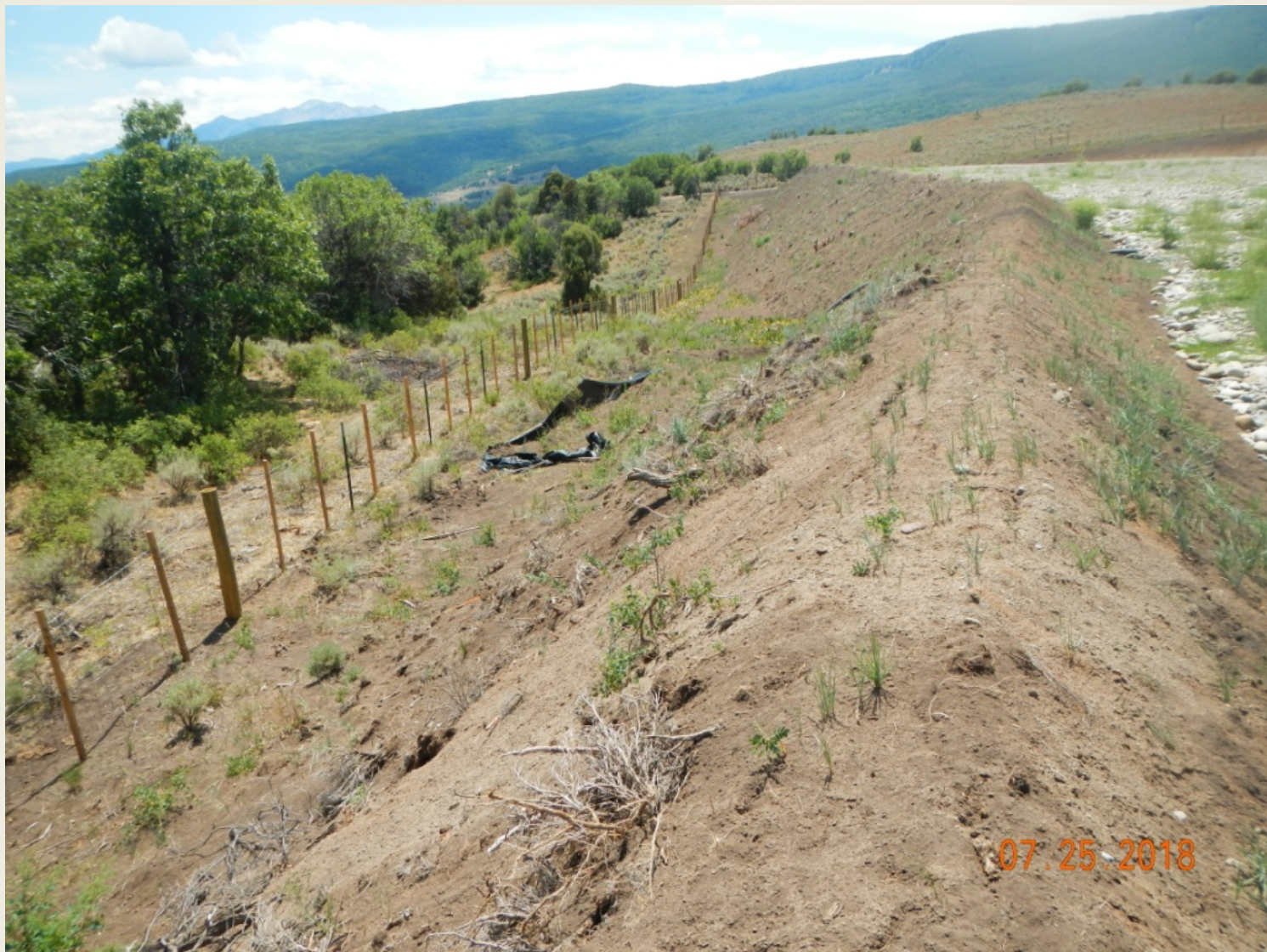
Photo 5. View of the southern portion of the project area from the southeastern corner facing northward. Silt fence is in disrepair.
