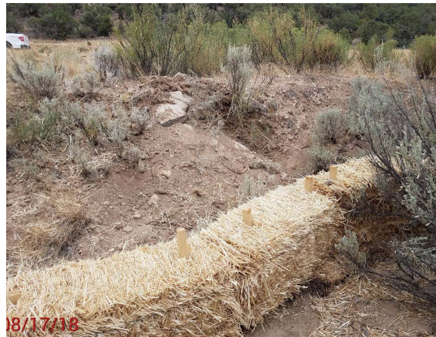
Location Photo #2, Storm water issue on lower berm resolved.
