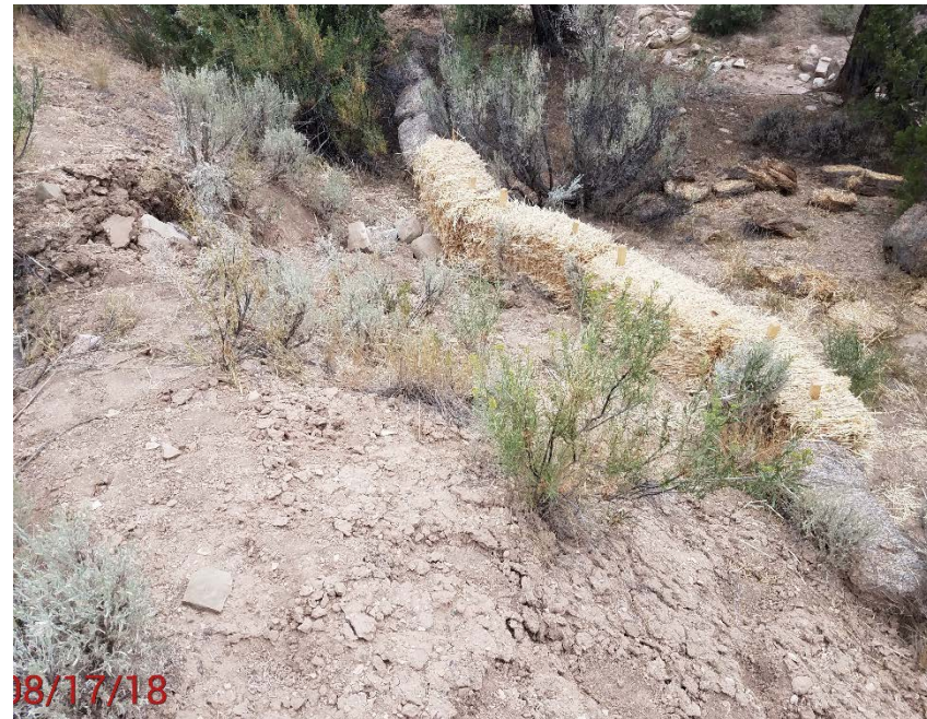
Location Photo #4, Strom water issue resolved on lower berm resolved.
