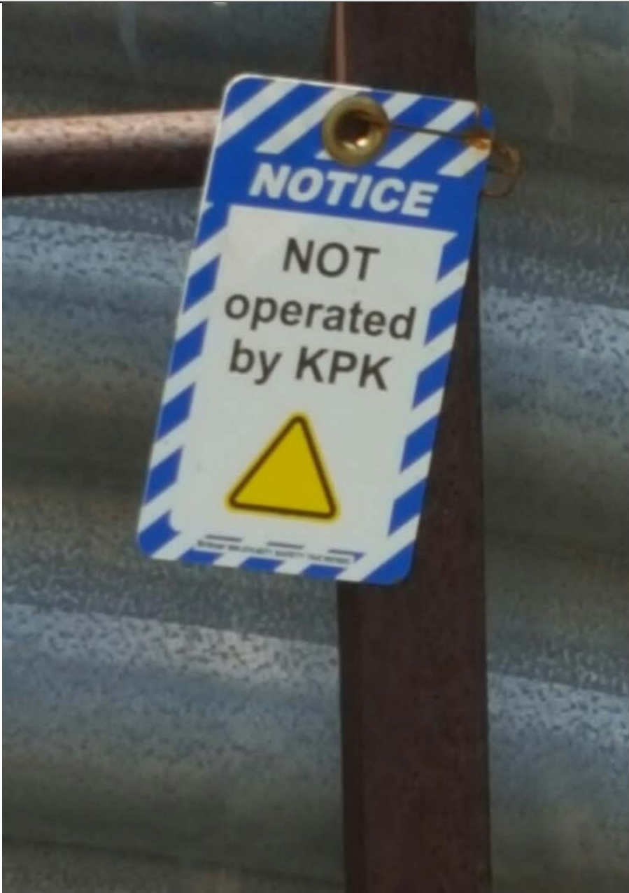
Figure #3 Risers have been tagged out.
