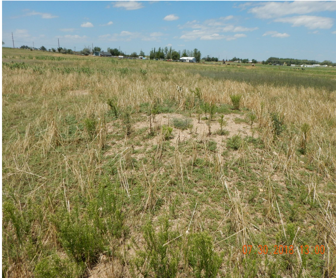
Photo 2. Photo taken from the western location, facing West. Operator has not contoured a portion of the location to match the surrounding landscape. Also, the photo illustrates vegetative standards do not meet Rule 1004 standards.
