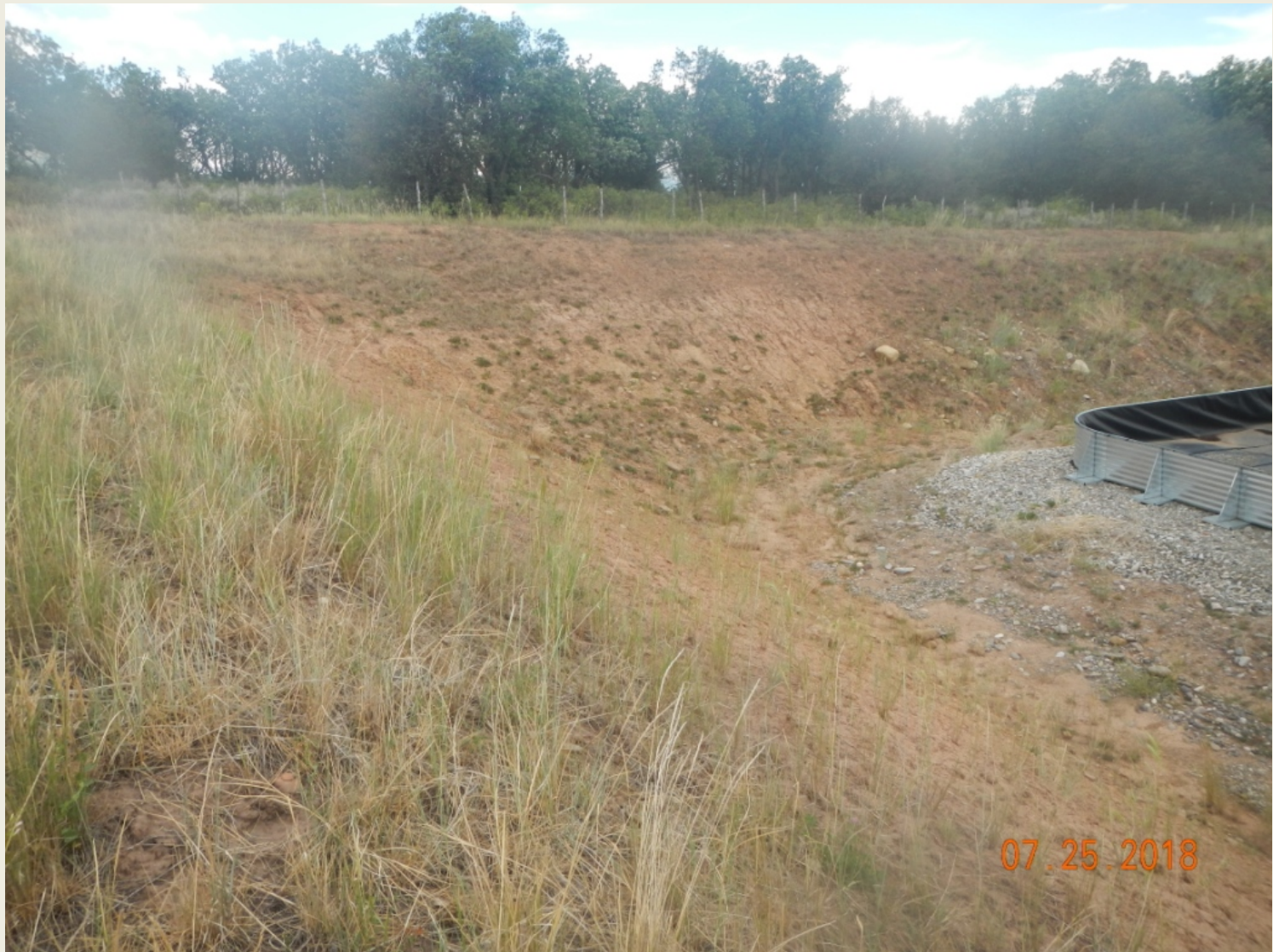
Photo 4. View of the northeastern cut-slope. Vegetation is progressing, but rilling is occurring here.
