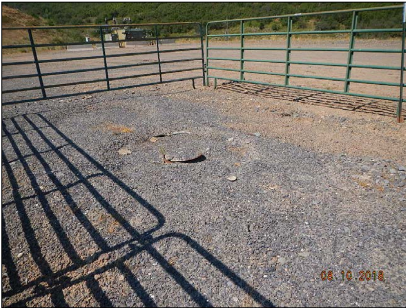
Photo 1. Top of conductors believed to be related to AL well.
