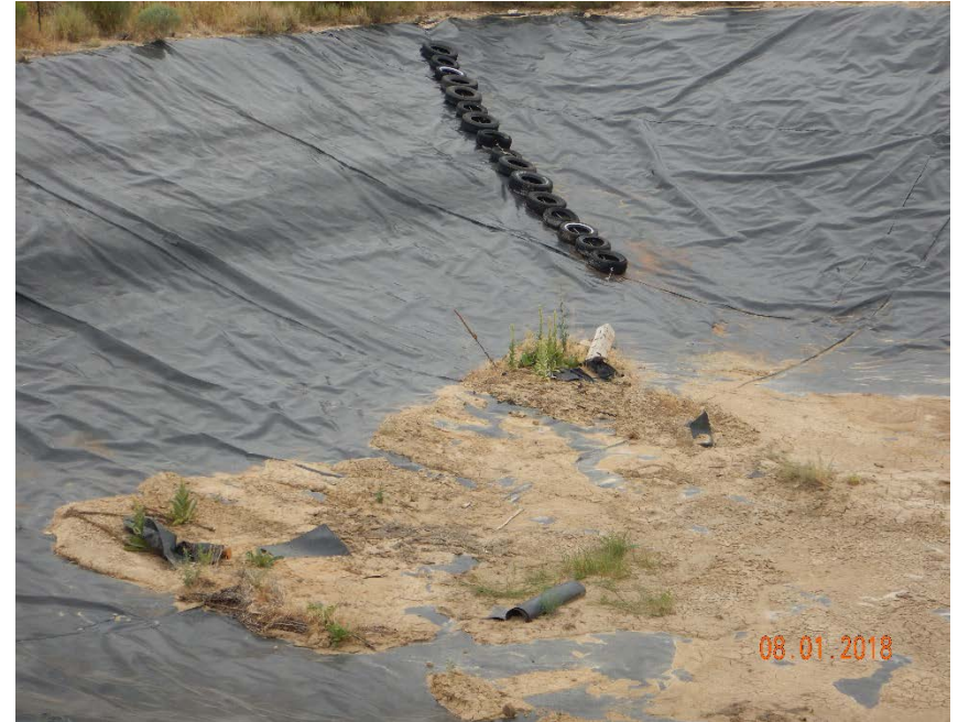
Photo #10 – Wood debris, vegetation, and scraps of liner located inside of pit.
