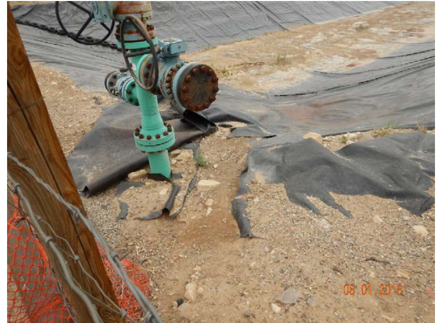
Photo #4 – Damaged pit liner, liner debris, and pipeline riser located at SW corner of pit.
