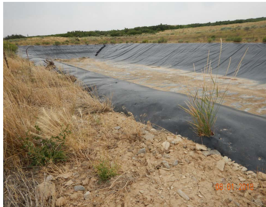
Photo #8 – Holes (and vegetation) in pit liner along anchor trench (4).
