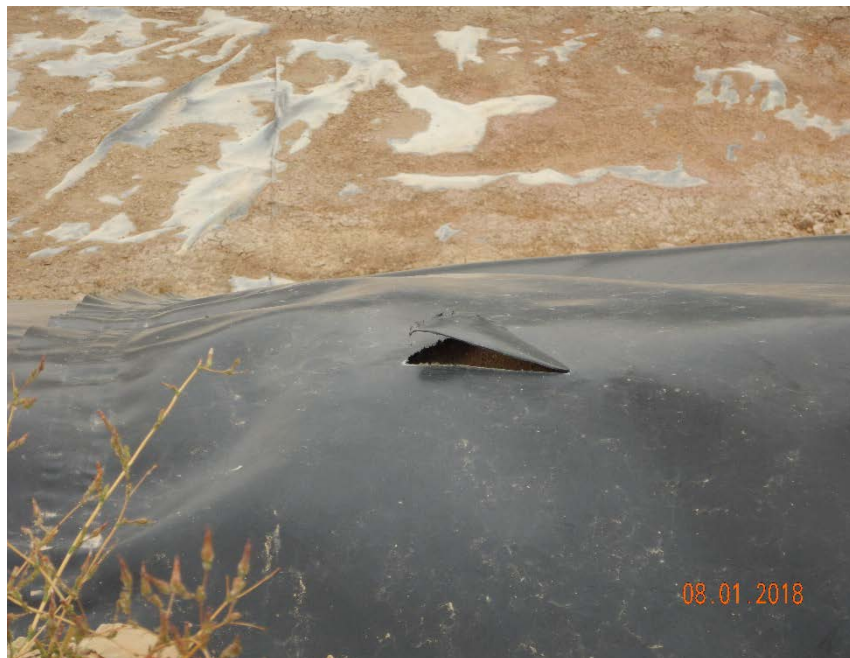
Photo #7 - Holes in pit liner along anchor trench (3).
