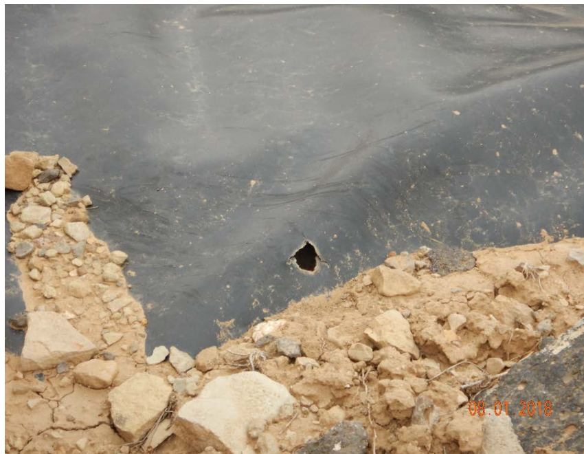
Photo #5 – Holes in pit liner along anchor trench (1).
