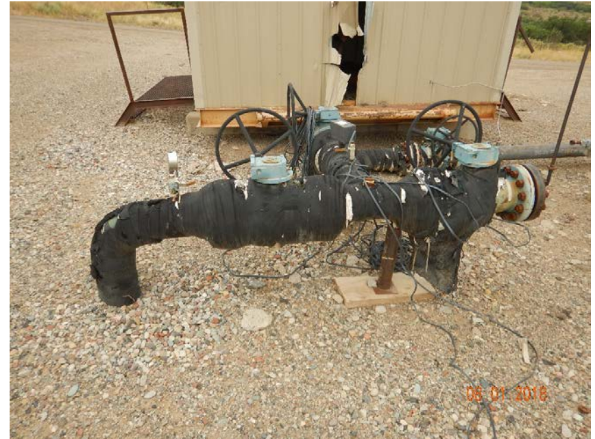
Photo #2 – Damaged shed and insulated flowline manifold located at SW corner of pit. Note tangled wiring draped on top of flowline manifold.
