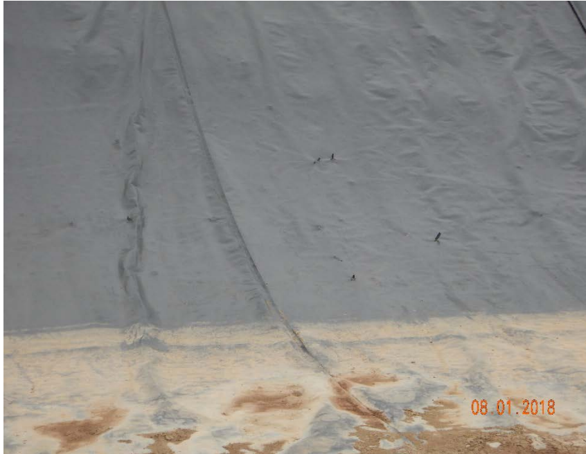
Photo #9 – Holes observed in pit liner along base of pit.
