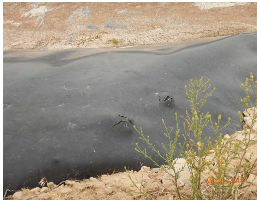
Photo #6 - Holes in pit liner along anchor trench (2).
