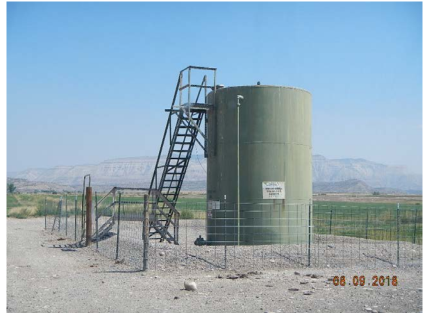
Photo 4. Tank with earth containment.
