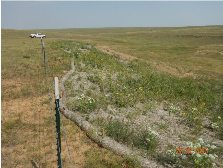
Photo 1: Photo taken from the southwest of the location, facing north. Photo shows vegetation on location appears to be progressing, and stormwater and erosion control BMPs appear to be in proper functioning condition.
