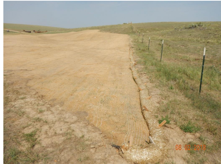
Photo 8: Photo taken from the east end of the fenced disturbance area, facing northwest. Photo shows reclamation work conducted. Disturbed areas appear to have been re-contoured/regraded. Erosion control blankets have been implemented and appear to have been installed in accordance to good engineering practices. Straw wattles have been installed on sections of the perimeter.
