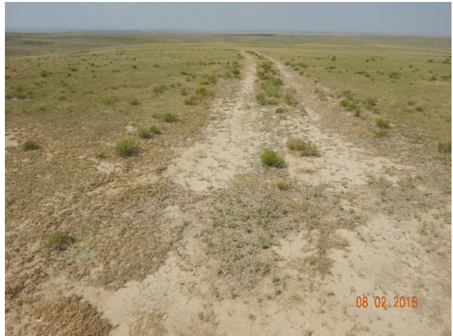
Photo 4: Photo taken from the west end of the location, facing southwest. Photo shows no reclamation activities, including compaction alleviation, recontouring/regrading and revegetation appear to have been conducted on the access road.
