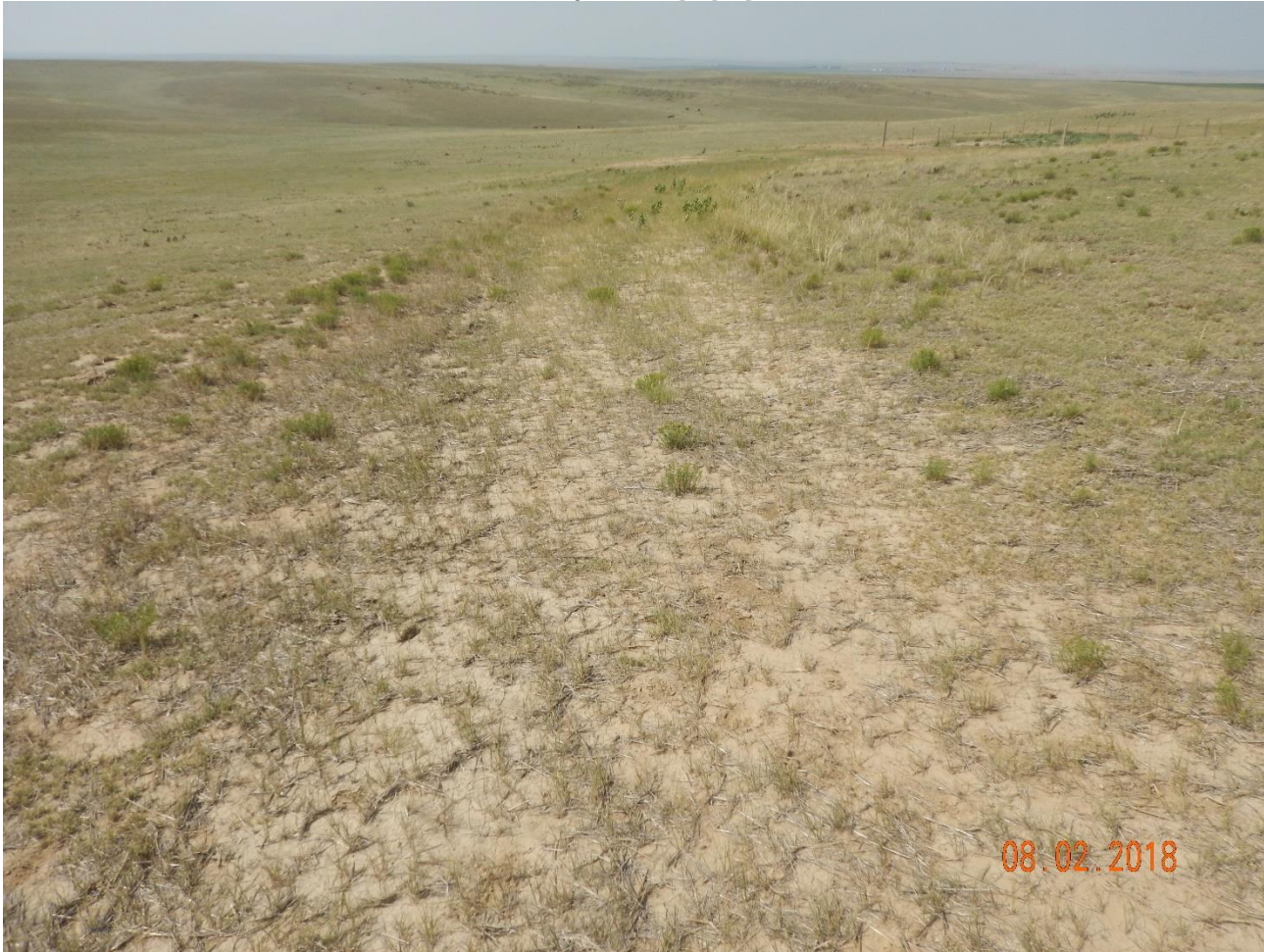
Photo 5: Photo taken from the east end of the location, facing southwest. Photo shows no reclamation activities, including compaction alleviation, recontouring/regrading and revegetation appear to have been conducted on the access road.
