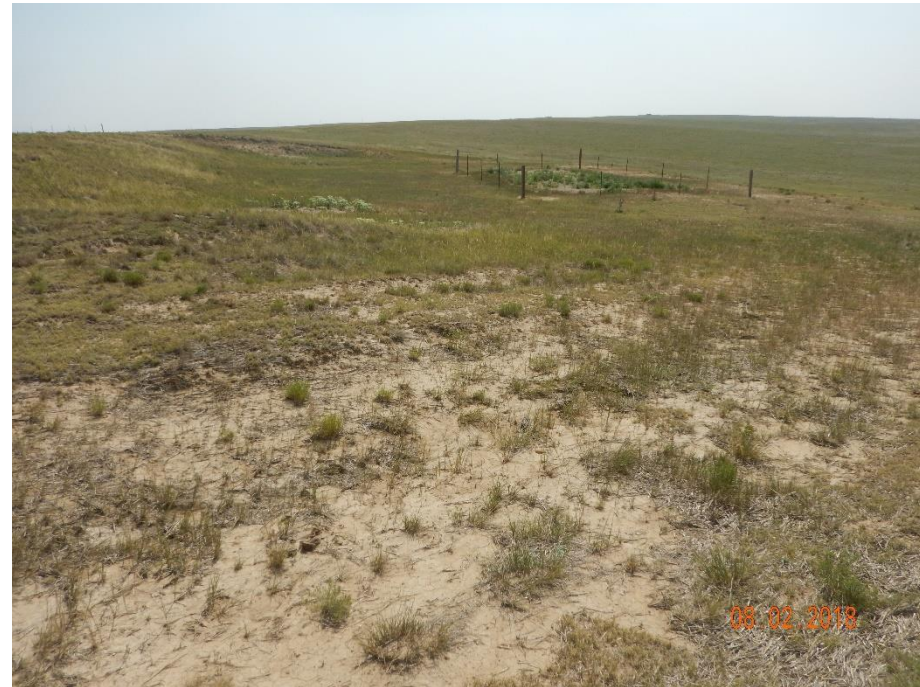
Photo 6: Photo taken from the west end of the location, facing southeast. Photo shows no reclamation activities, including compaction alleviation, recontouring/regrading and revegetation appear to have been conducted on the access road.
