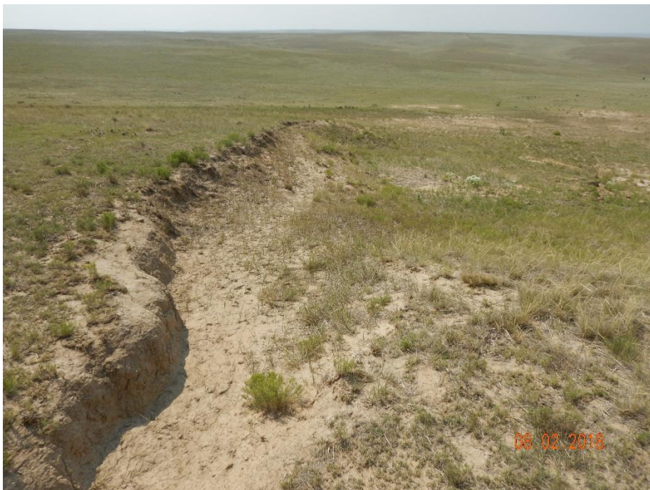
Photo 1: Photo taken from the northeast corner of the location, facing south. Photo shows erosion degradation on the location. Photo also shows the location has not be recontoured/regraded in accordance to 1004.a
