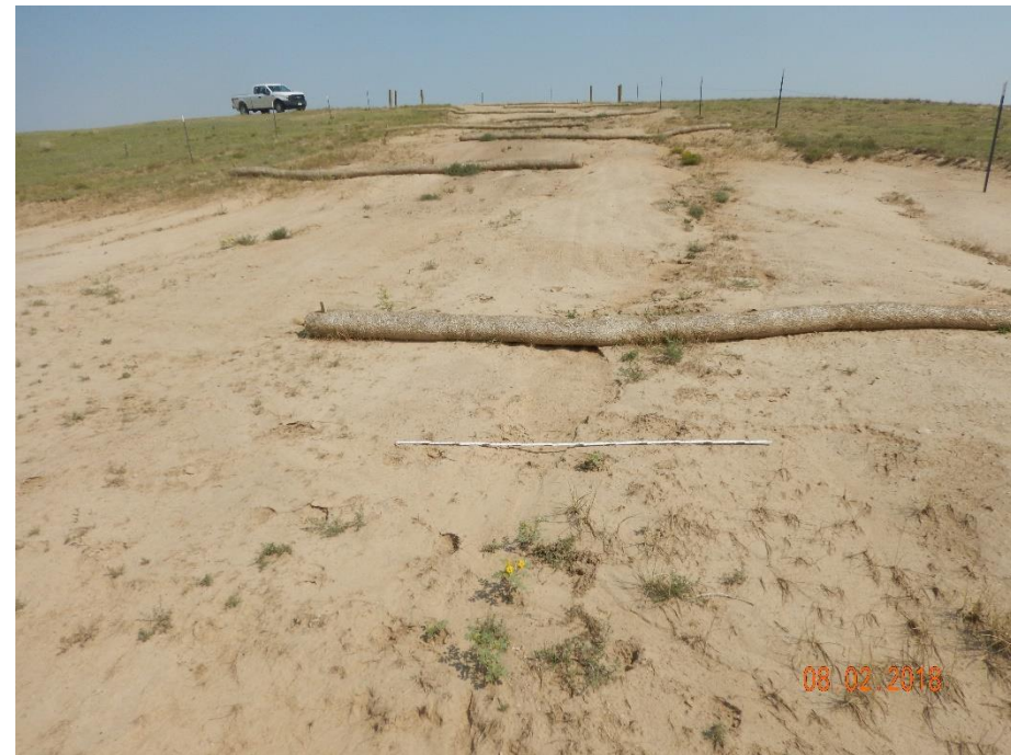
Photo 6: Photo taken from the location, facing north. Photo shows that straw wattles improperly installed and insufficient, and that stormwater erosion has been allowed to continue. See comments under photo 1. Six (6) foot measuring stick for reference.
