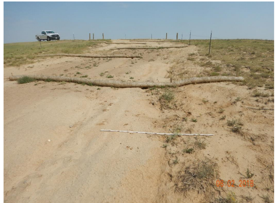
Photo 4: Photo taken from the location, facing north. Photo shows that straw wattles improperly installed and insufficient, and that stormwater erosion has been allowed to continue. See comments under photo 1. Six (6) foot measuring stick for reference.
