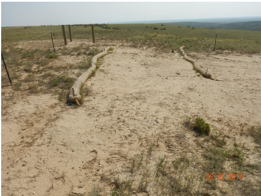
Photo 1: Photo taken from the northwest end of the fenced spill area facing east. Previous inspections required operator to perform reclamation and stormwater management (properly select and install site specific stormwater and sediment control BMPs). Reclamation activities were previously conducted, however it was documented that no controls to stabilize the seeded soil were implemented per the corrective action, and that the seeded soil was at risk to wind and stormwater erosion. Photo shows that straw wattles improperly installed and insufficient, and that stormwater erosion has been allowed to continue. Additionally, photo also shows that vegetation has failed to germinate and establish on the location.
