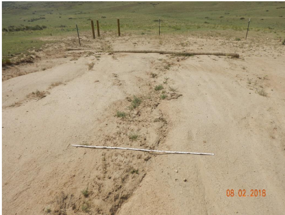
Photo 5: Photo taken from the location, facing south. Photo shows that straw wattles improperly installed and insufficient, and that stormwater erosion has been allowed to continue. See comments under photo 1. Six (6) foot measuring stick for reference.
