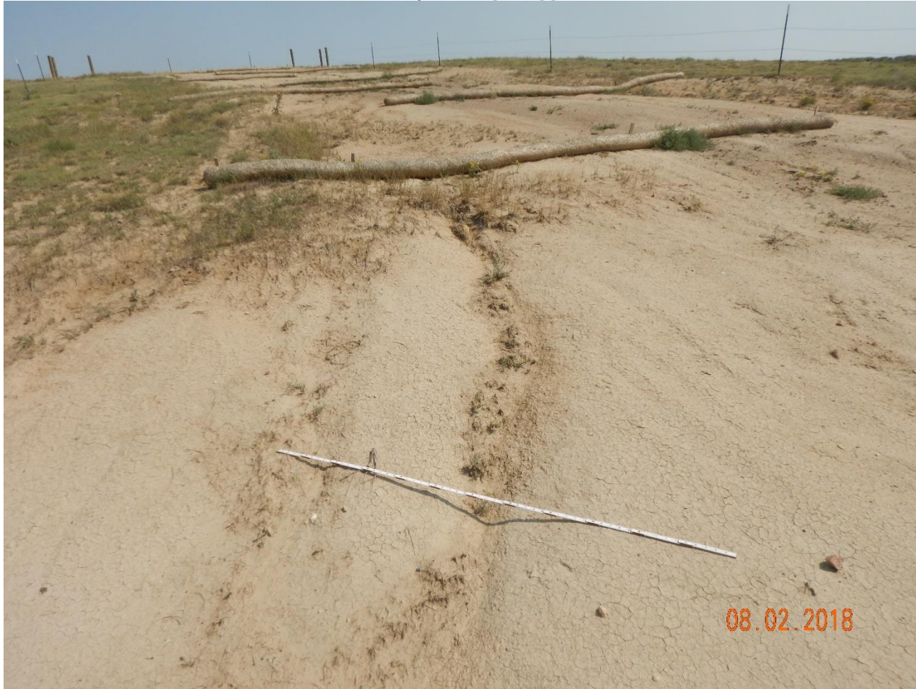
Photo 5: Photo taken from the location, facing north. Photo shows that straw wattles improperly installed and insufficient, and that stormwater erosion has been allowed to continue. See comments under photo 1. Six (6) foot measuring stick for reference.
