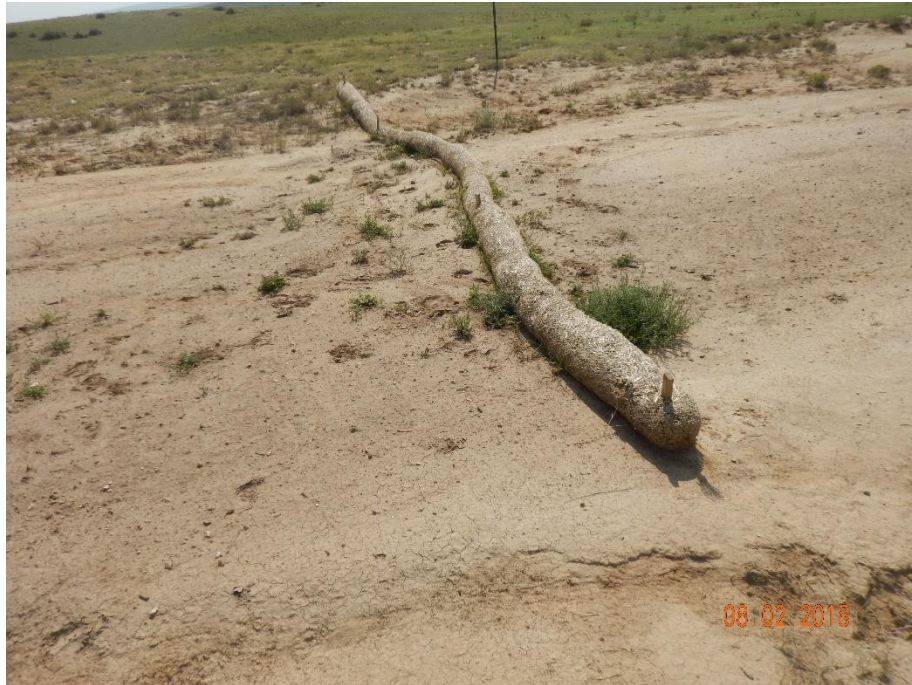
Photo 3: Photo taken from the location. Photo shows that straw wattles improperly installed and insufficient, and that stormwater erosion has been allowed to continue. See comments under photo 1.
