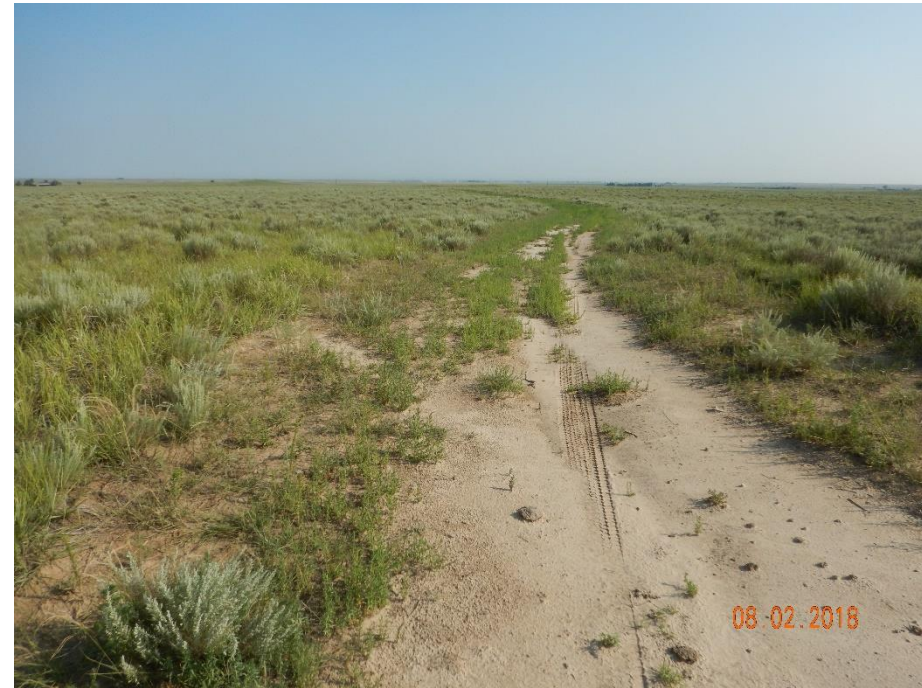
Photo 2: Photo taken from the location facing north. Photo shows access road. Access road has not been recontoured/regraded, and remains either bare and exposed soil, or vegetation is predominantly undesirable weedy plant species. Unable to find evidence of additional reclamation activities have been conducted.
