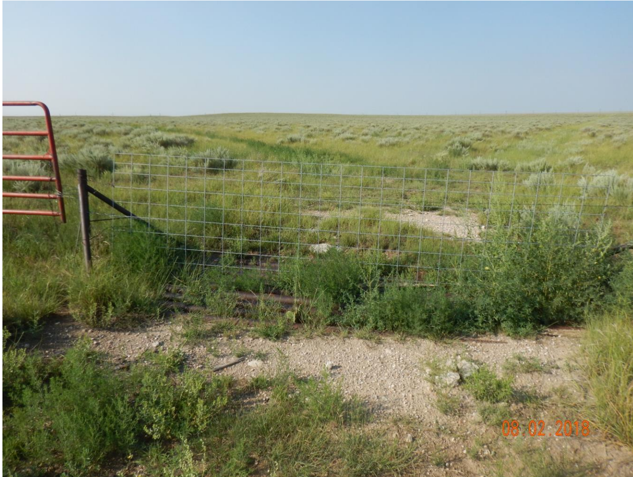
Photo 3: Photo taken at access road entrance. Photo shows surface owner appears to have constructed a panel across the cattle guard to prevent access. Cattle guard requires removal in accordance to COGCC 1000 series reclamation requirements.
