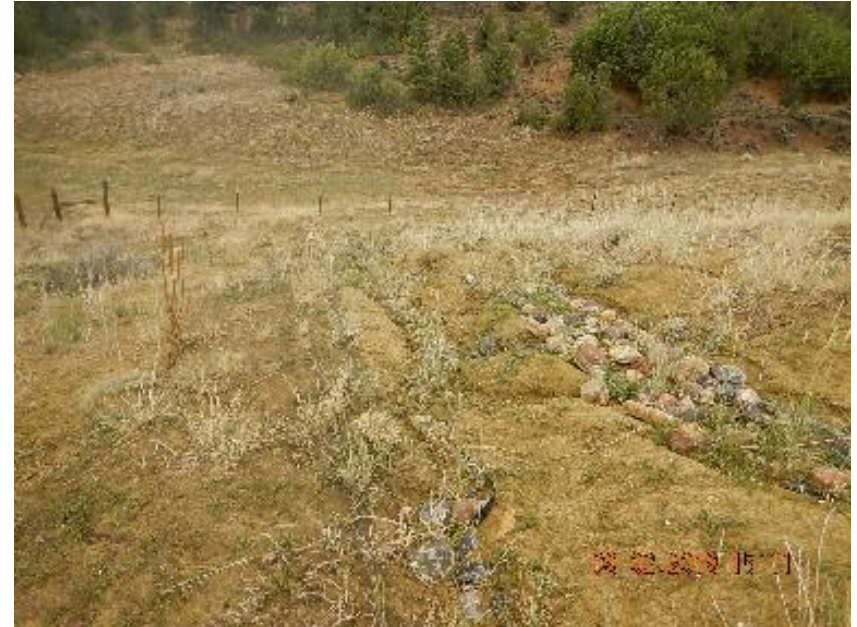
Photo 6: Fill slope erosion on SE corner of location.
