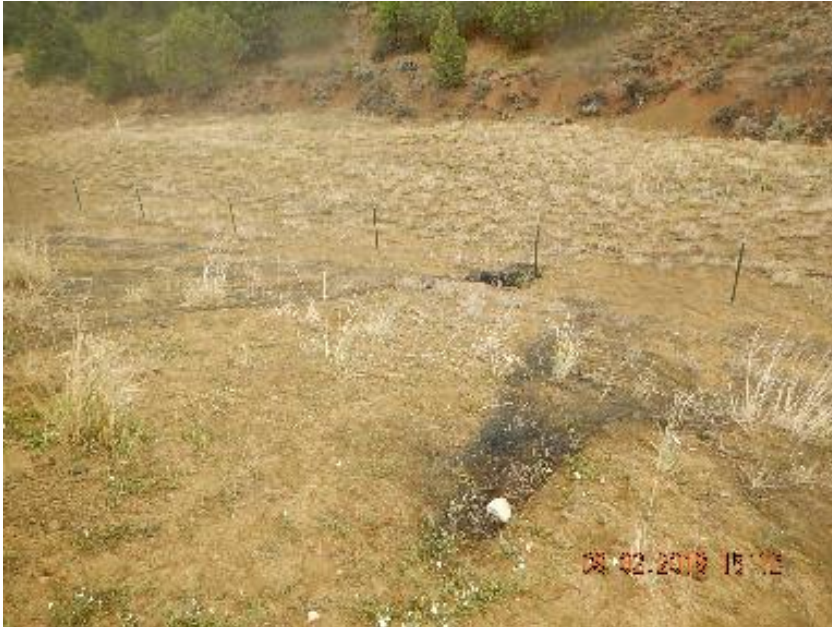
Photo 5: Loose blanket material on fill slope .
