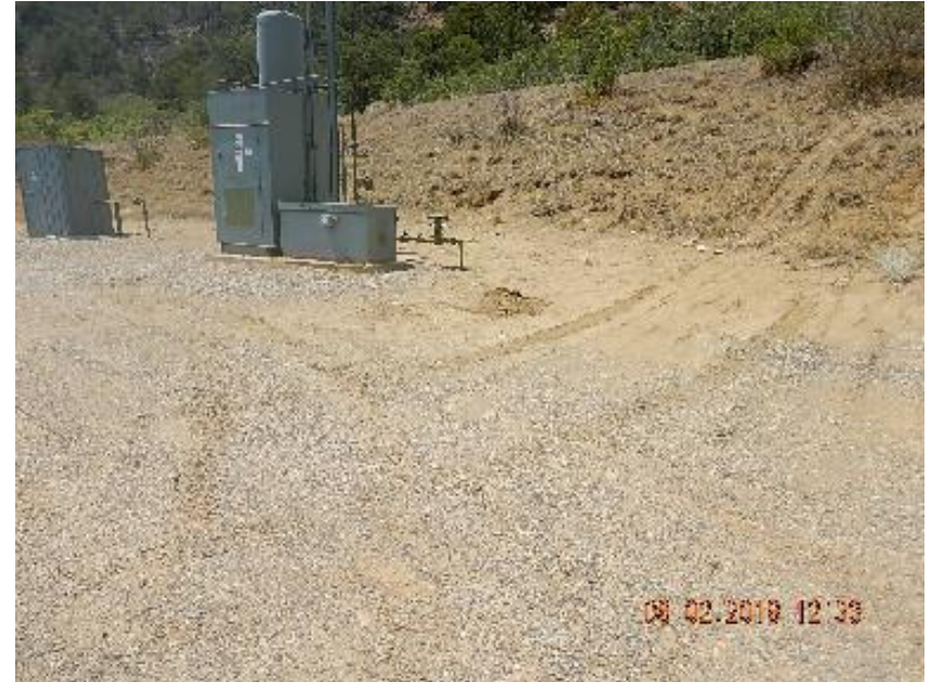
Photo 4: Sediment flow onto location from cut slope.
