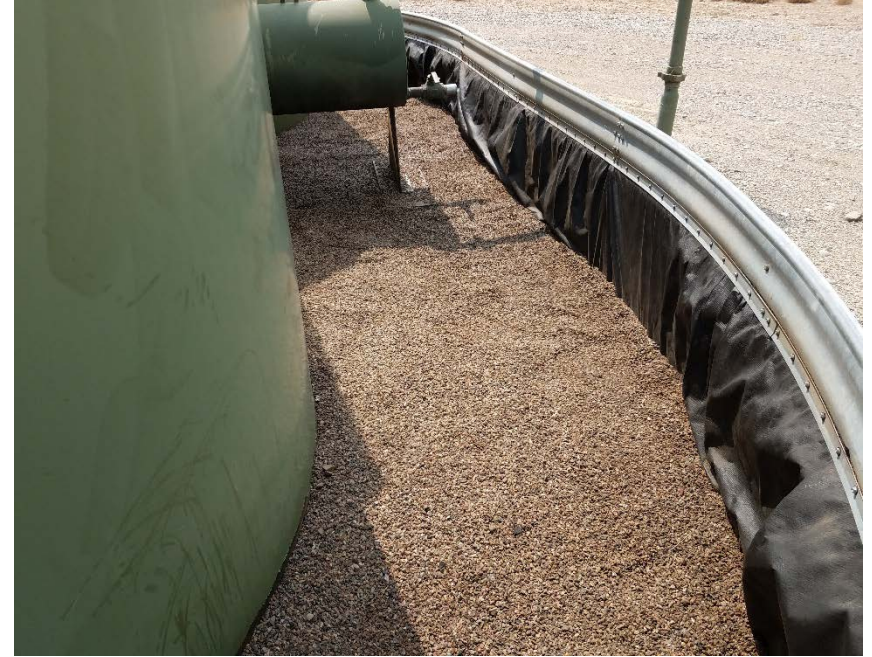
Location Photo #6, Stained rock in battery containment.
