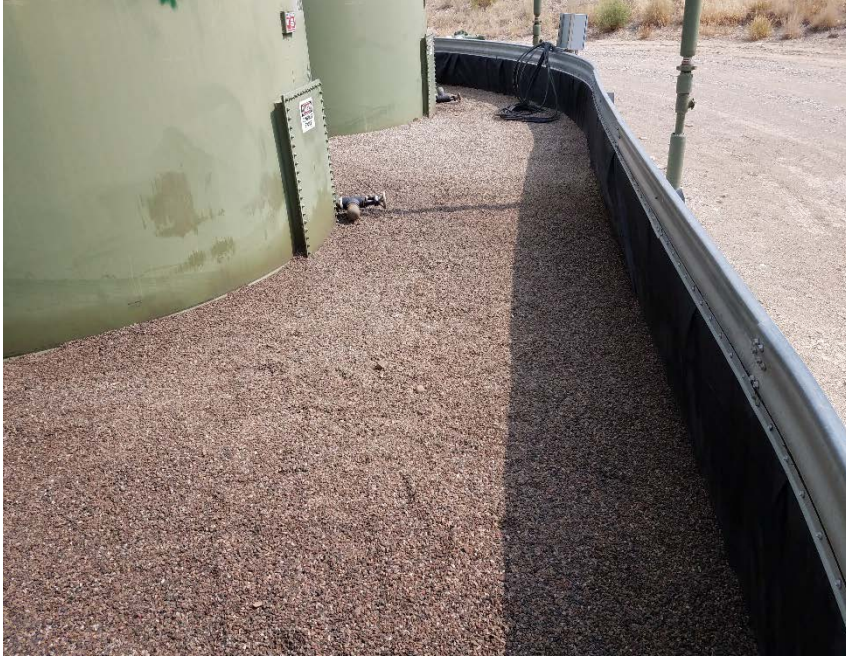
Location Photo #3, stained rock in battery containment.
