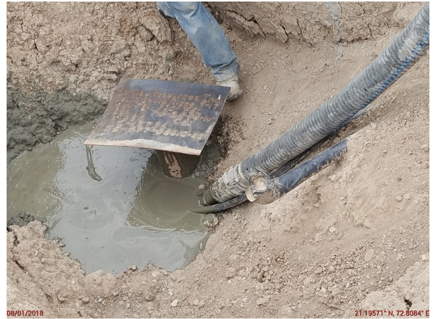
Photo 2. Plate placed on well after cement to surface.
