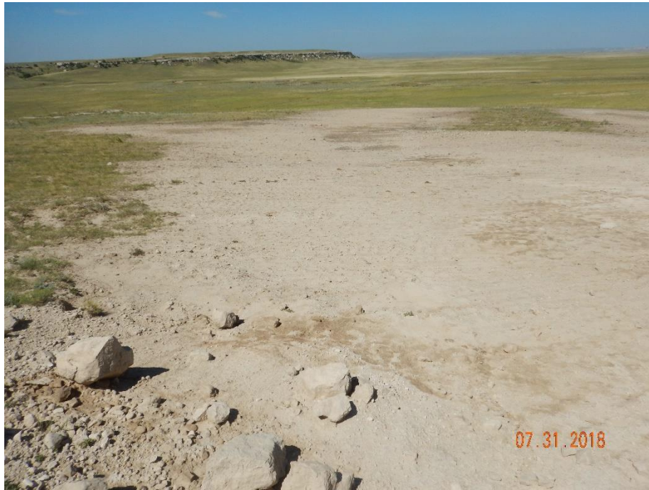
Photo 13: Photo taken from the southwest corner of the pit, facing west. Photos show interim areas of the south and east of the pit have been regraded and appears to have been reseeded. However, no stabilization or stormwater and erosion control BMPs have been installed per the corrective actions
