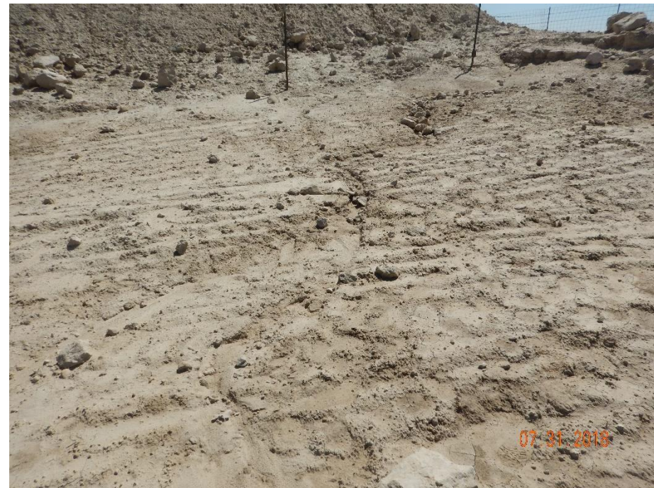
Photo 14: Photo shows operator appears to have regraded and reseeded the disturbance areas. However, no stabilization or stormwater and erosion control BMPs have been installed per the corrective actions. Photos show erosion degradation has been allowed to re-occur on the slope.
