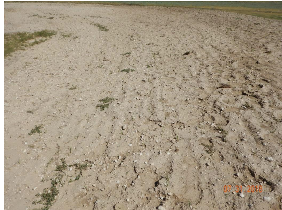
Photo 4: Photo taken from the central interim areas of the location (see photos 1-2). Photos show interim areas of the location have been regraded and appears to have been reseeded. However, no stabilization or stormwater and erosion control BMPs have been installed per the corrective actions.
