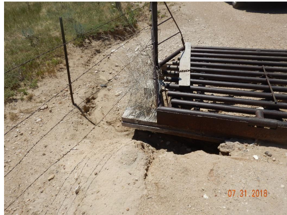
Photo 16: Photo taken from the access road gate, north of the location facing south. Photo shows stormwater erosion has cut underneath the cattle guard. This needs to be repaired and stabilized.
