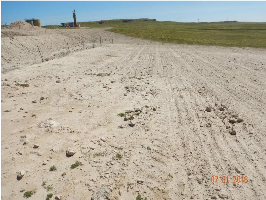
Photo 11: Photo taken from the southwest corner of the pit, facing south. Photos show interim areas of the south and east of the pit have been regraded and appears to have been reseeded. However, no stabilization or stormwater and erosion control BMPs have been installed per the corrective actions
