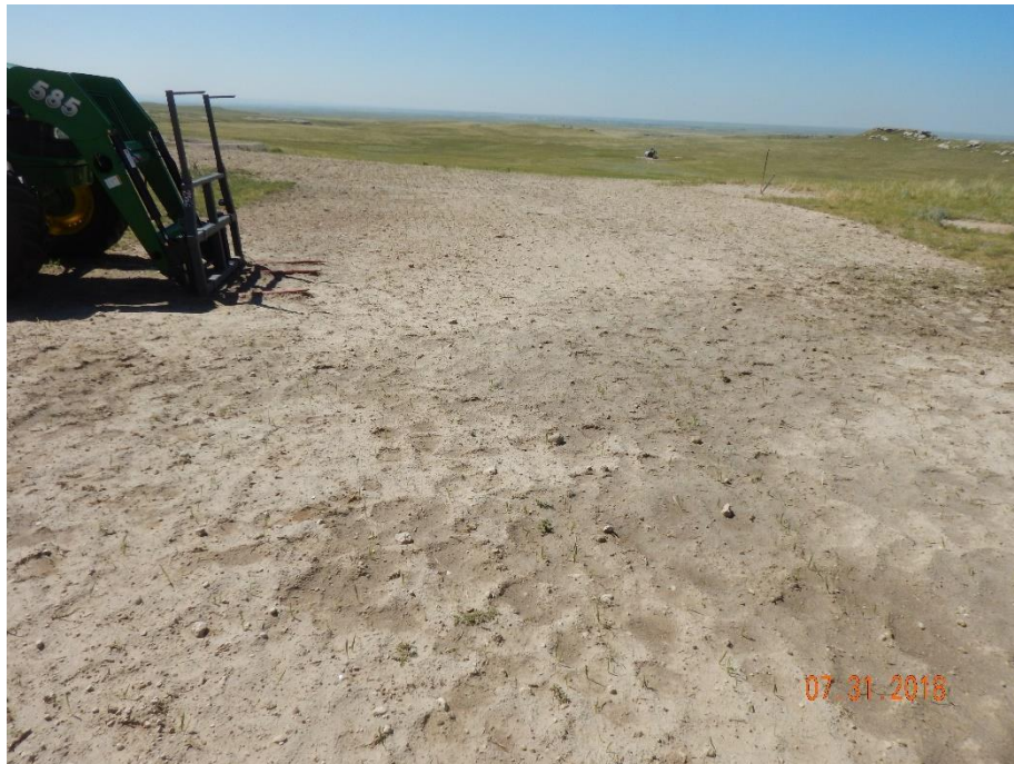
Photo 5: Photo taken from the south end of the location, facing south. Photos show interim areas of the location have been regraded and appears to have been reseeded. However, no stabilization or stormwater and erosion control BMPs have been installed per the corrective actions.
