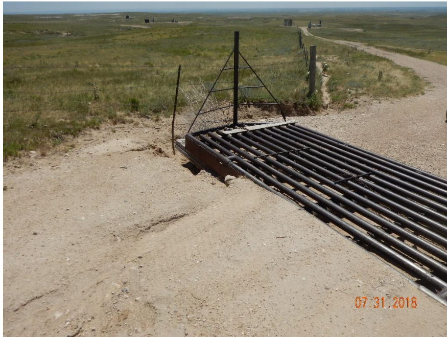
Photo 15: Photo taken from the access road gate, north of the location facing south. Photo shows stormwater erosion has cut underneath the cattle guard. This needs to be repaired and stabilized.
