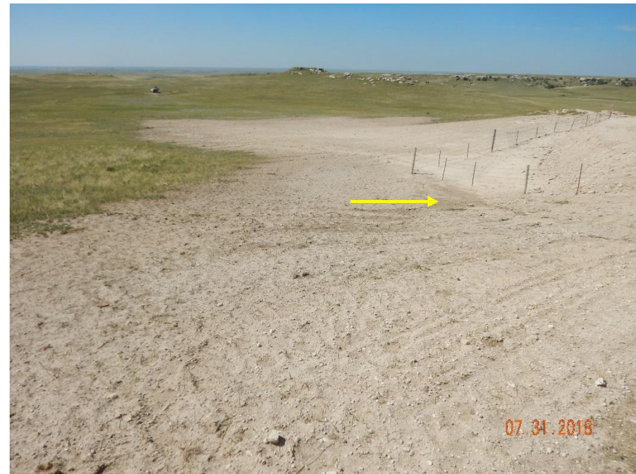
Photo 6: Photo taken from the south end of the location, facing southwest. Photos show interim areas of the south and east of the pit have been regraded and appears to have been reseeded. However, no stabilization or stormwater and erosion control BMPs have been installed per the corrective actions. Photos show erosion degradation has been allowed to continue on the slope.
