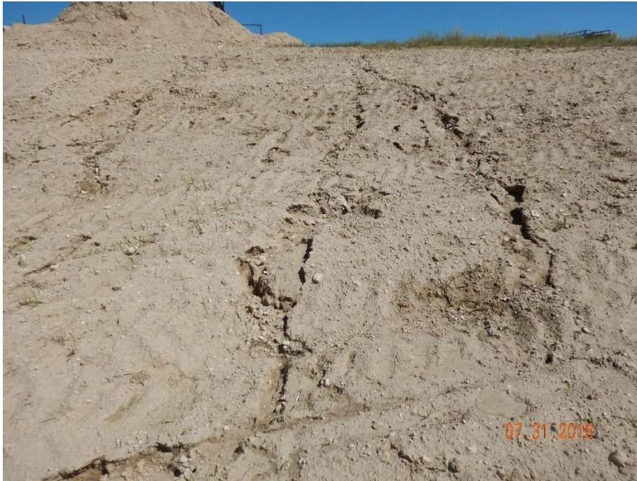
Photo 7: Continued from photo 6. Photo taken from the slopes east of the pit, facing south. Photo shows operator appears to have regraded and reseeded the disturbance areas. However, no stabilization or stormwater and erosion control BMPs have been installed per the corrective actions. Photos show erosion degradation has been allowed to continue on the slope.
