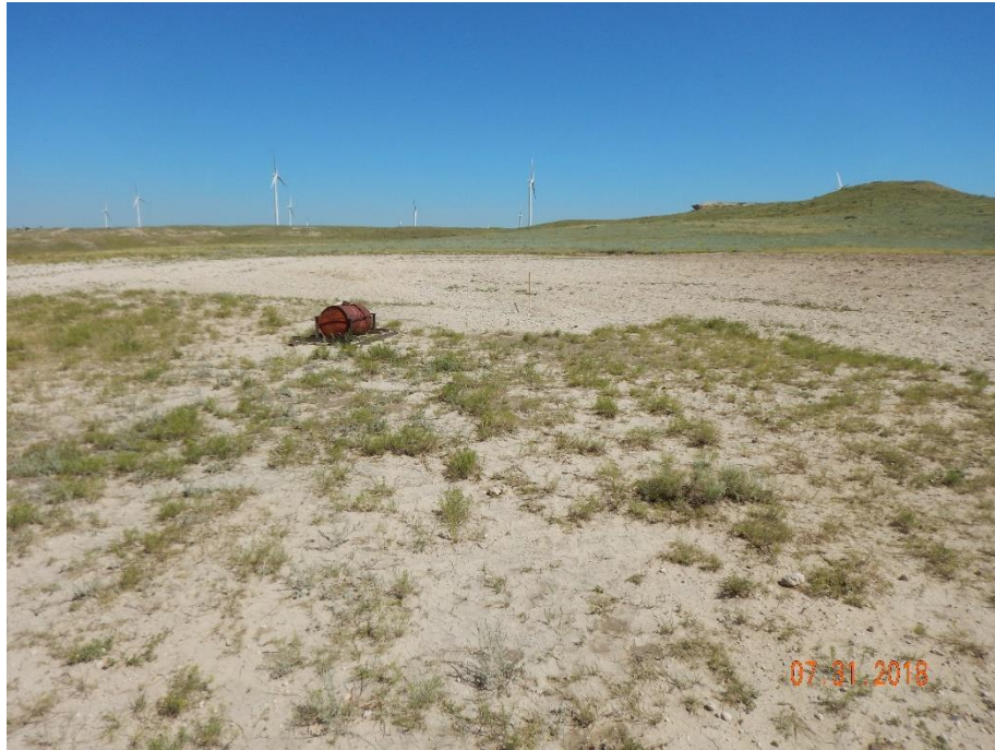
Photo 1: Photos 1-2 taken from the northeast end of the pumpjack, facing northeast to east. Photos show interim areas of the location have been regraded and appears to have been reseeded. However, no stabilization or stormwater and erosion control BMPs have been installed per the corrective actions.
