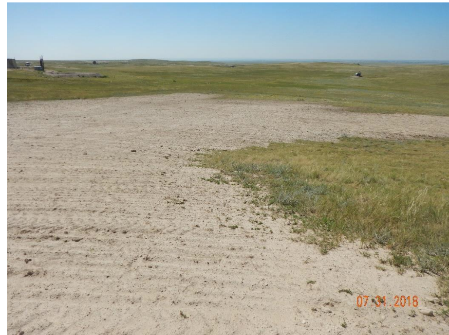
Photo 10: Photo taken from the southwest corner of the pit, facing south. Photos show interim areas of the south and east of the pit have been regraded and appears to have been reseeded. However, no stabilization or stormwater and erosion control BMPs have been installed per the corrective actions
