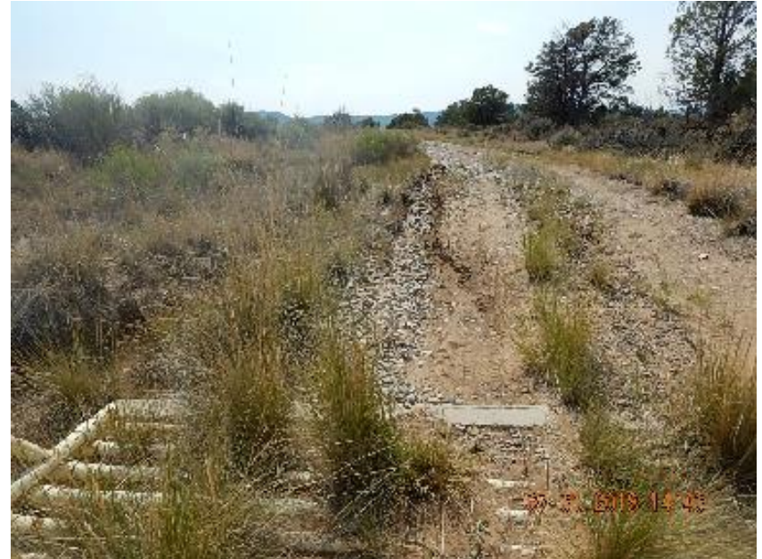
Photo 4: Erosion channel at wellhead pad entrance.
