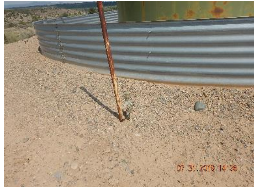
Photo 2: Unused 1" steel riser at production tank.
