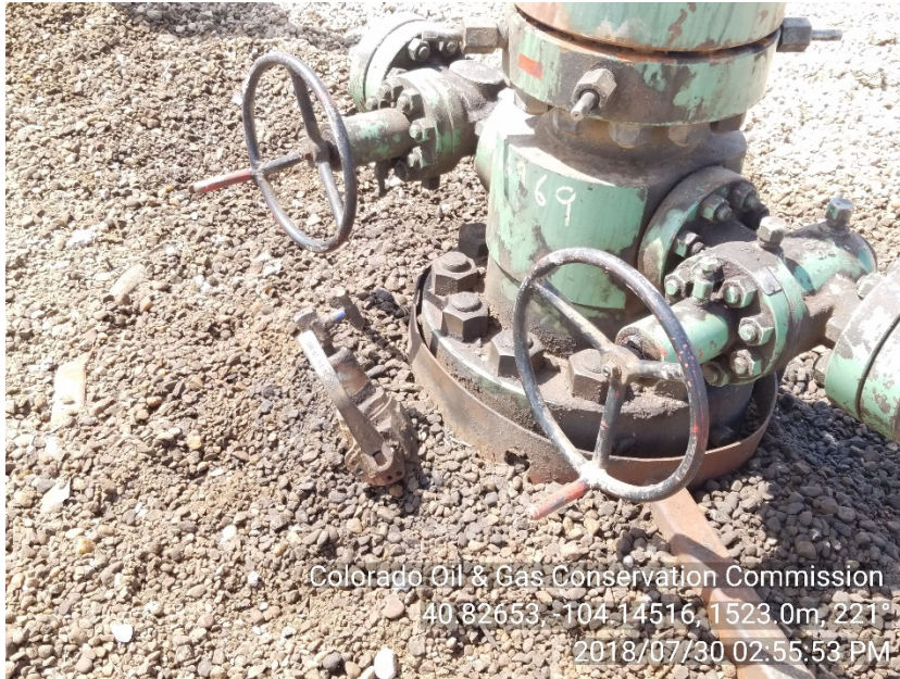
Photo #5 NGL C9B (API 05-123-40770) injection well Bradenhead
