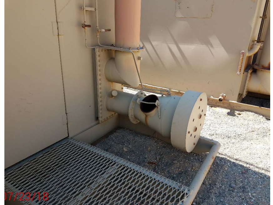
Location Photo #2, missing wildlife screen
