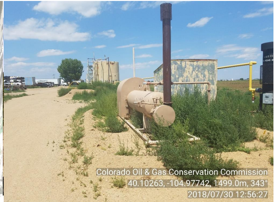
Photo 4. Separator Corrective actions: Control weeds around Headed separator.
