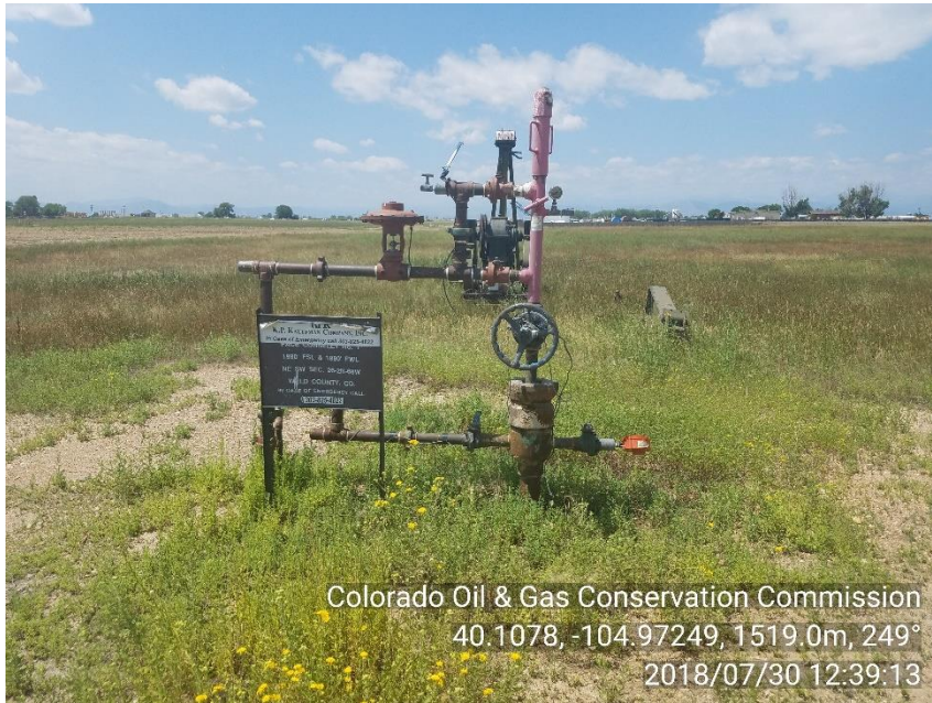
Photo 1. Wellhead Corrective actions: Control weeds at wellhead and lease road. Remove unused equipment (pumping unit).
