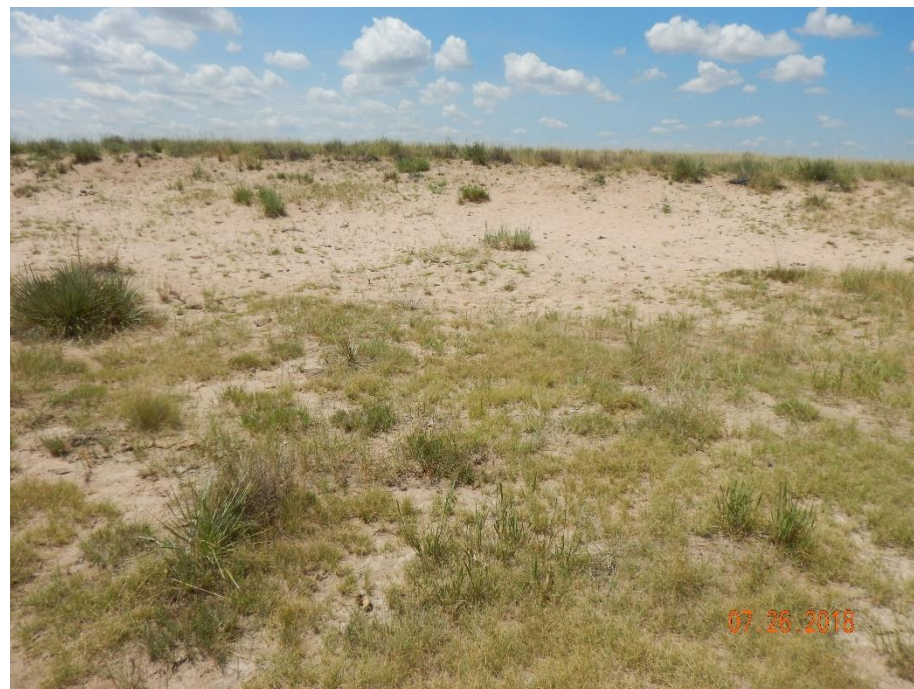
Photo 2: Photo taken from the location, facing southwest. Photo shows areas of the cut slope that remain predominantly bare and exposed soil. Additional reclamation and stabilization is required.
