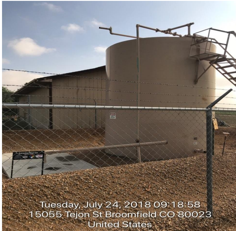
Photo#1 Production tank and produced water pit
