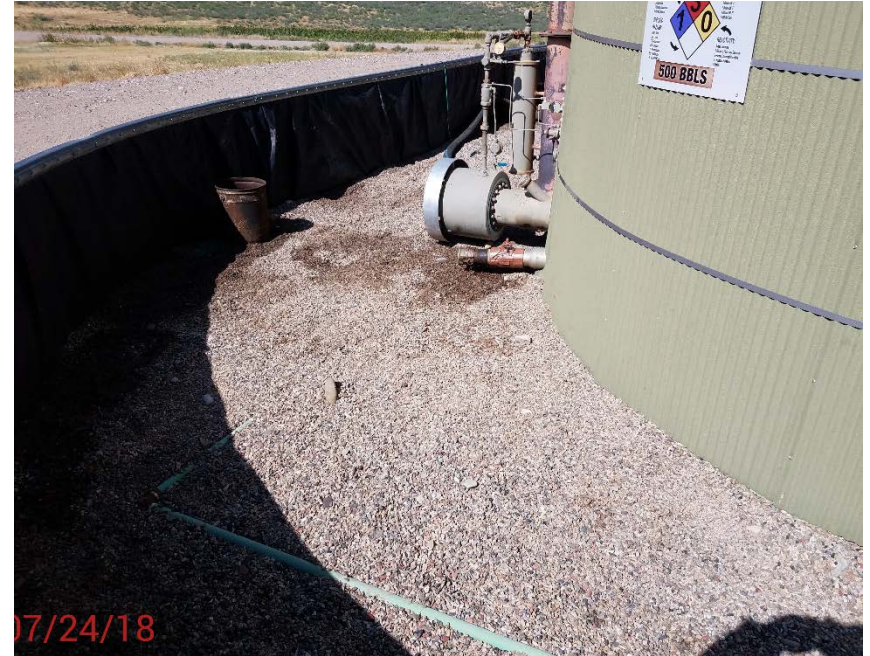
Location Photo #4, stained material in battery containment
