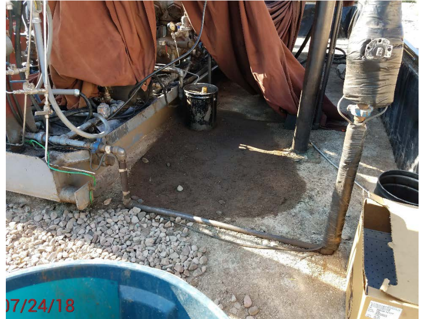
Location Photo #6, Stained material in compressor containment
