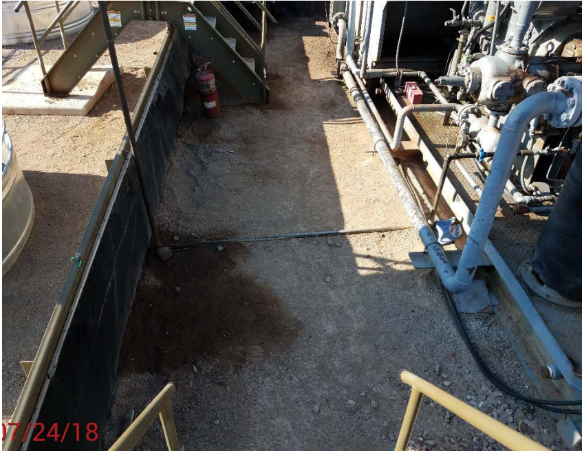
Location Photo #5, Stained material in compressor containment
