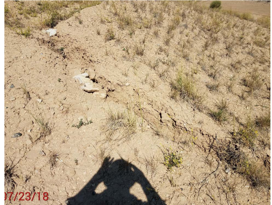
Location Photo #7, slope erosion in SW corner, midslope
