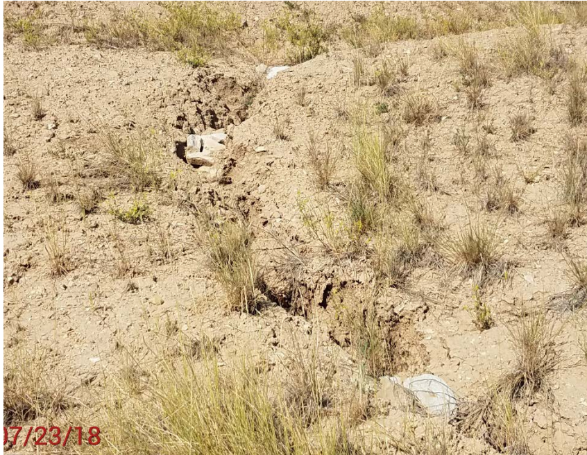
Location Photo #6, slope erosion in SW corner, midslope
