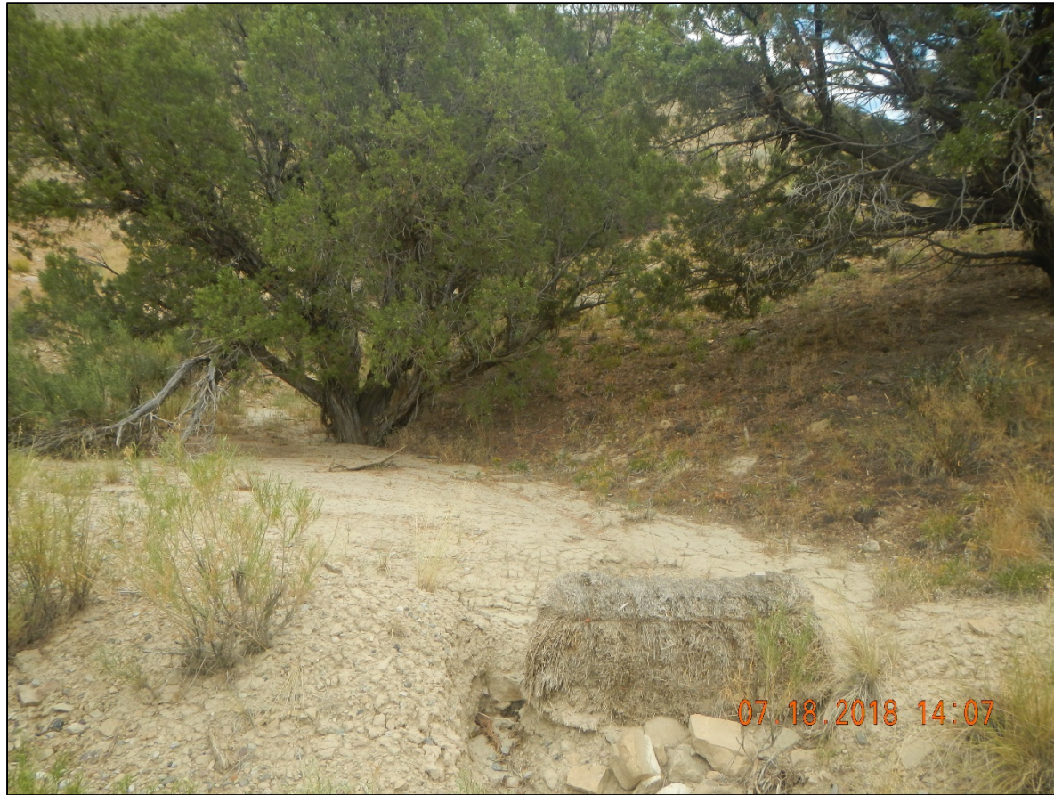
Sediment build up in check dam and washing around bale. 39.48180 -108.05495
