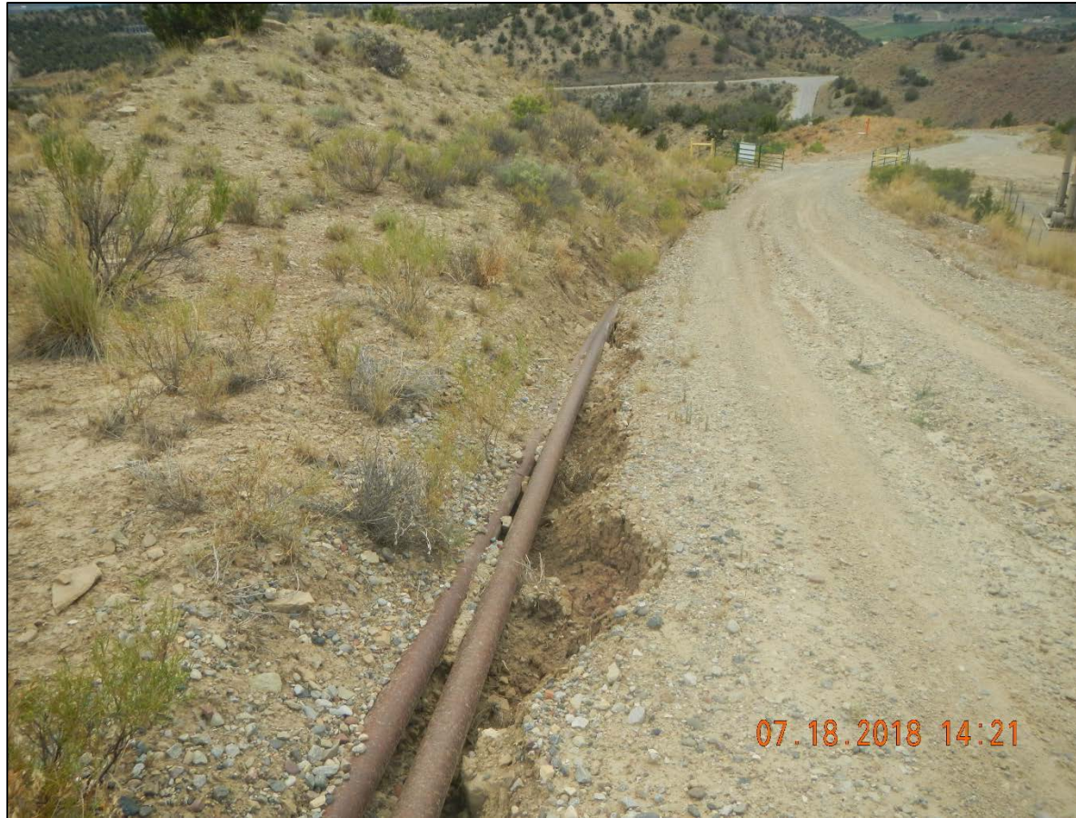
Erosion of road and ditch.
