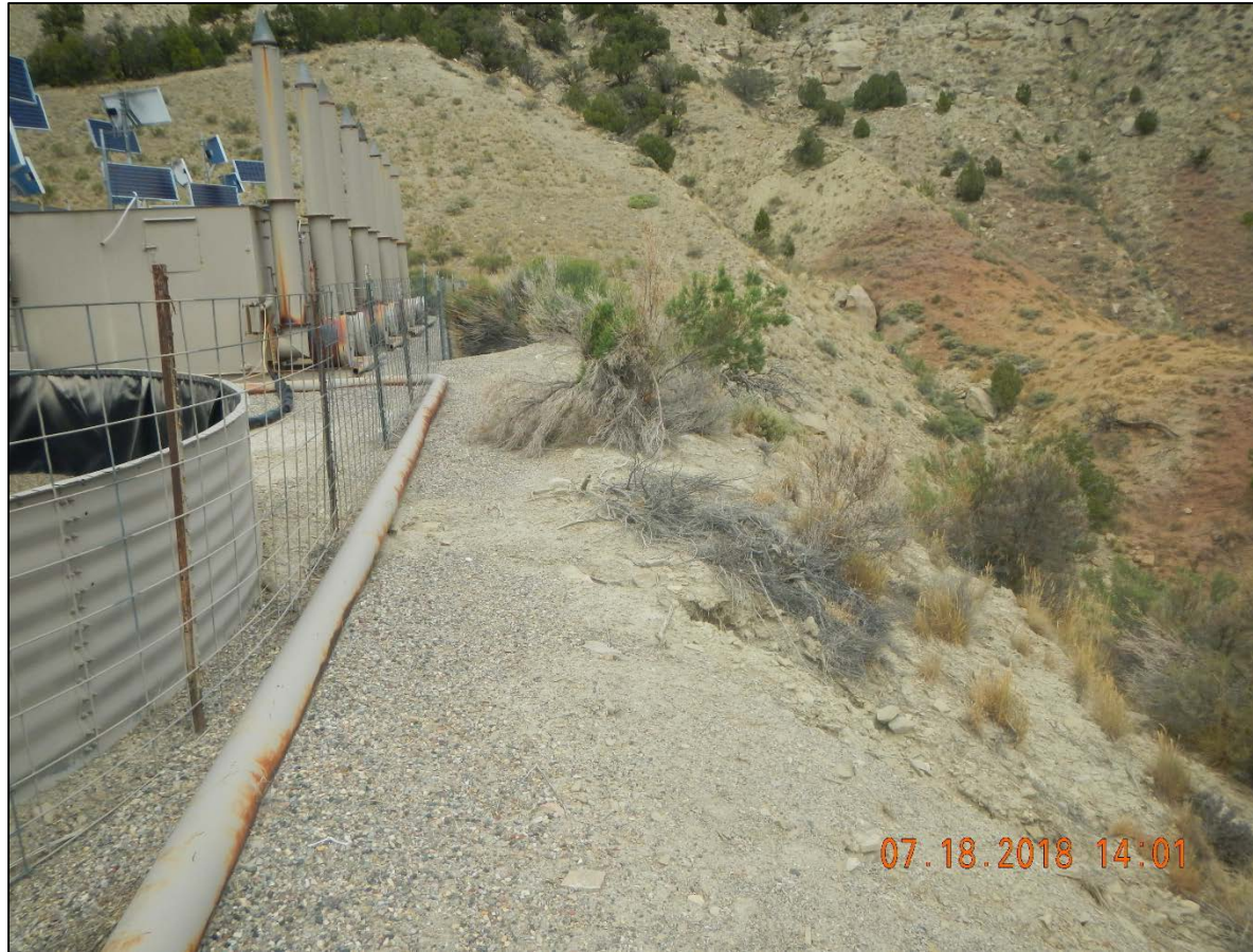
Erosion on edge of location behind separators.
