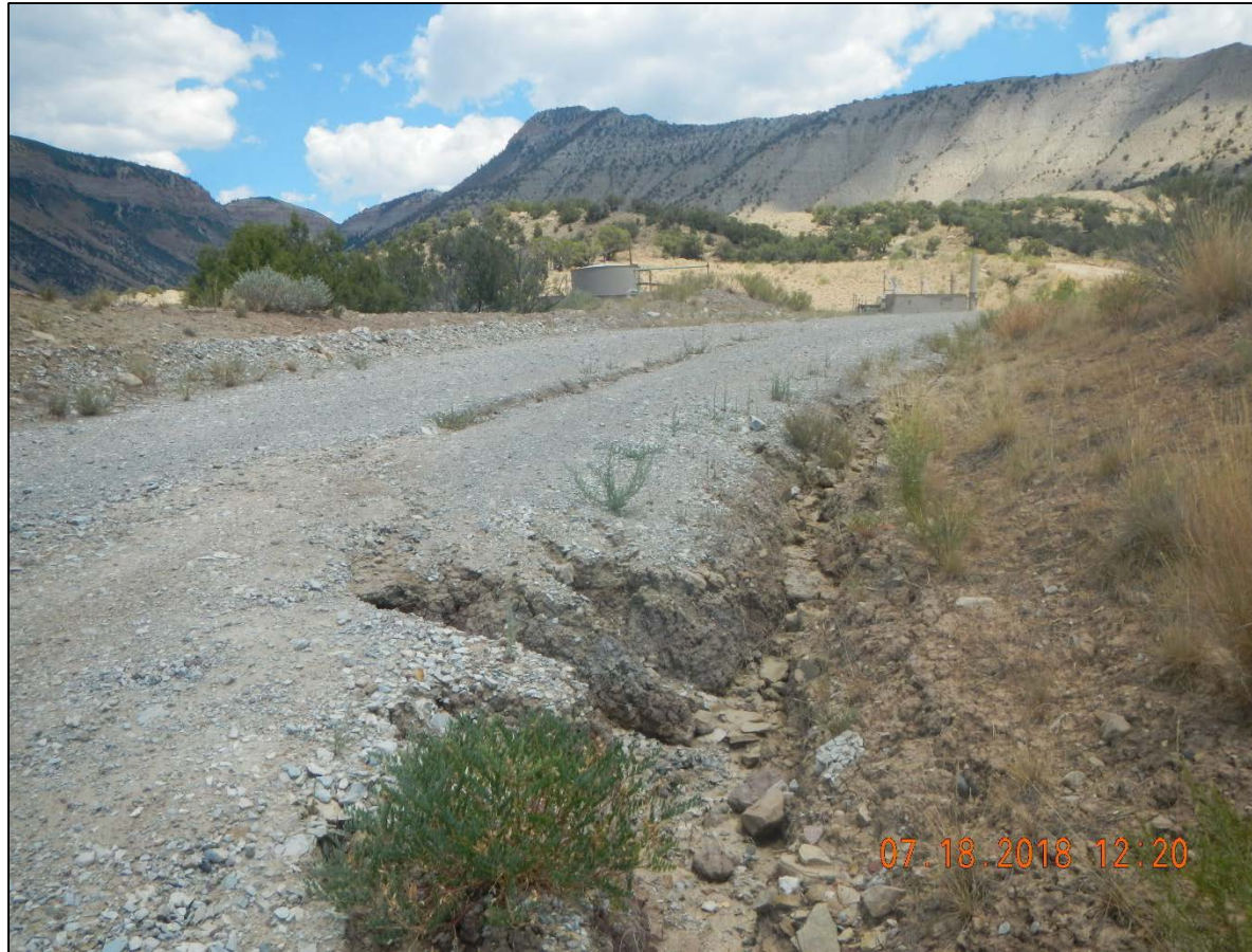
Washing of road into ditch. Near GM 23-36 location in the back ground.
