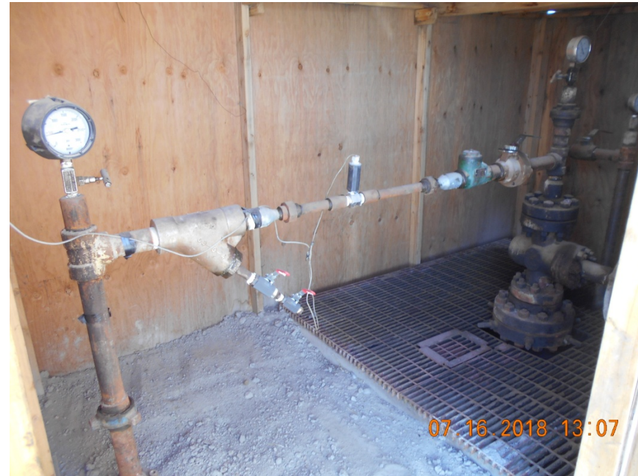
Injection wellhead inside housing
