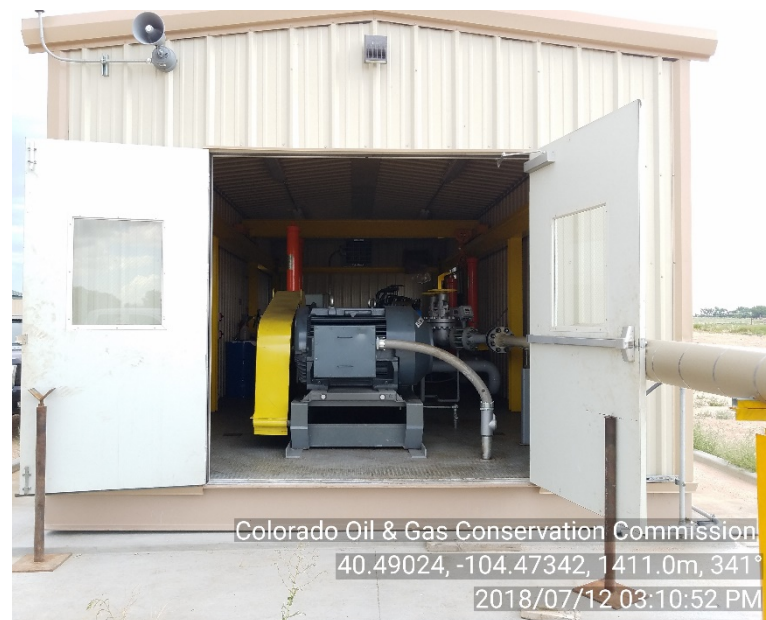
Photo #6 NGL Apollo 11 (API 05-123-42210) Injection pump
