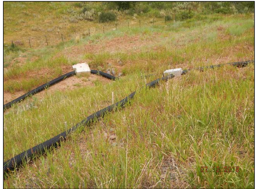
Photo 2. SW drains off fill slope.
