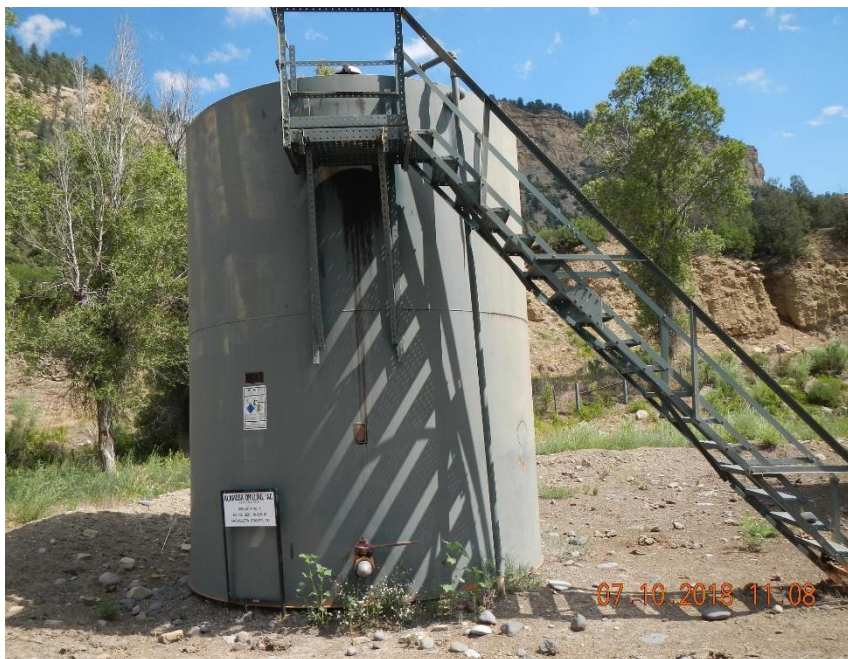
300 bbl. AST for Nielson #4 in shared earthen secondary containment berm with Albert Martinez #1 ASTs.
