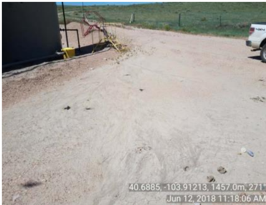
COGCC Photo 5: Stormwater erosion on NW side of location
