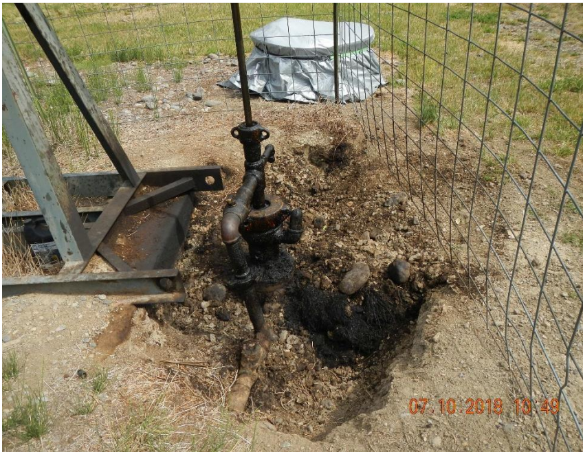
Removal of stained soil around well head has begun. Excavation is approximately 2' deep currently.
