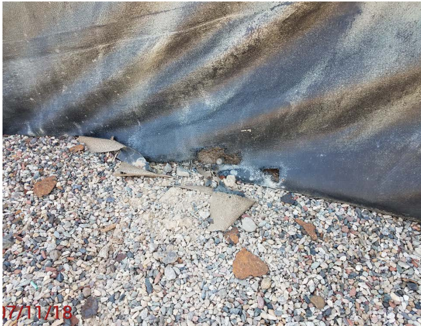
Location Photo #5, Holes in battery containment
