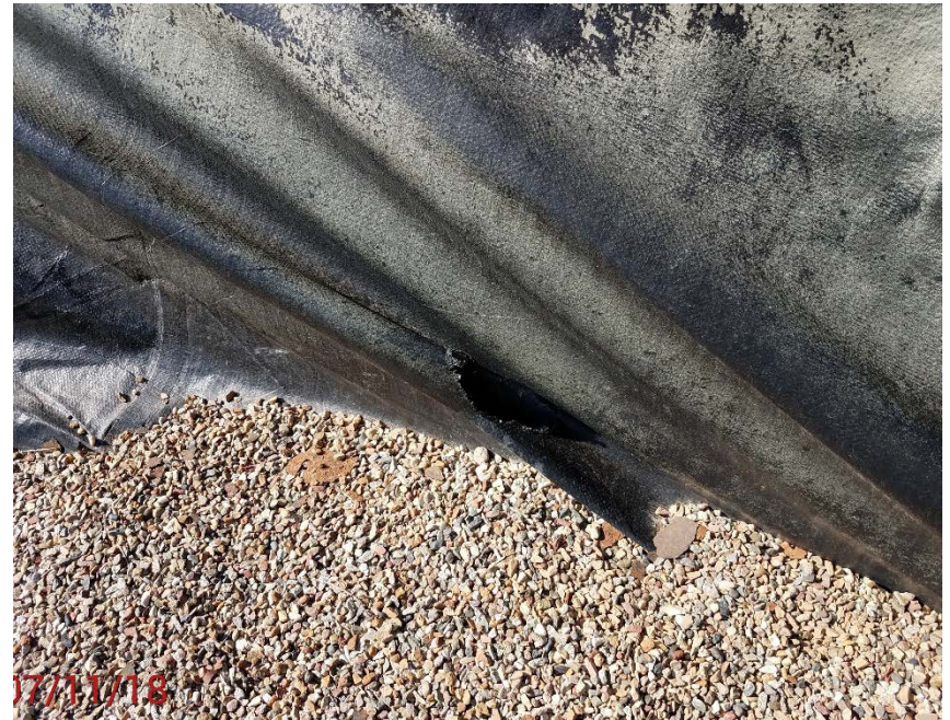
Location Photo #6 , Holes in battery containment
