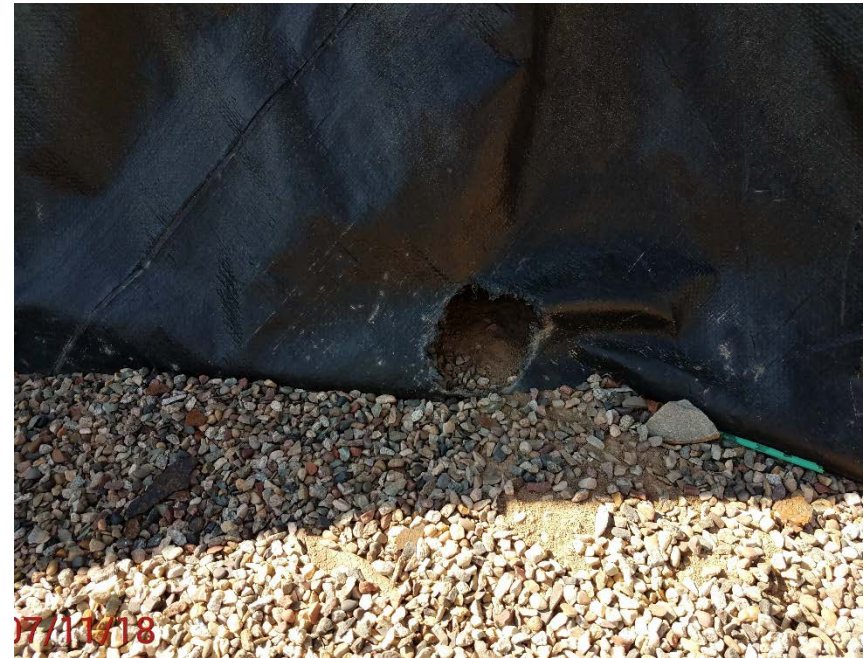
Location Photo #4, Holes in battery containment
