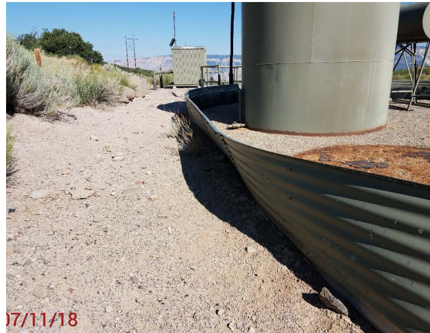
Location Photo #2, Containment wall maintenance
