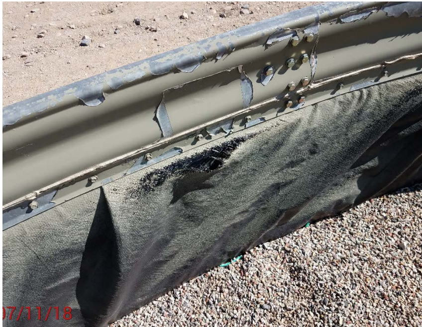
Location Photo #3, Holes in battery containment
