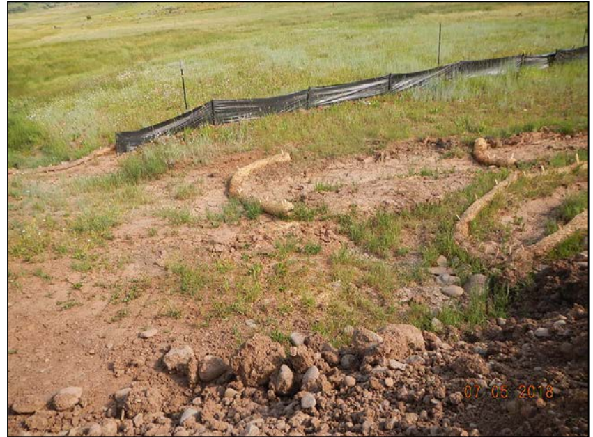
Photo 2. Irrigation water no longer bypassing stormwater BMPs.
