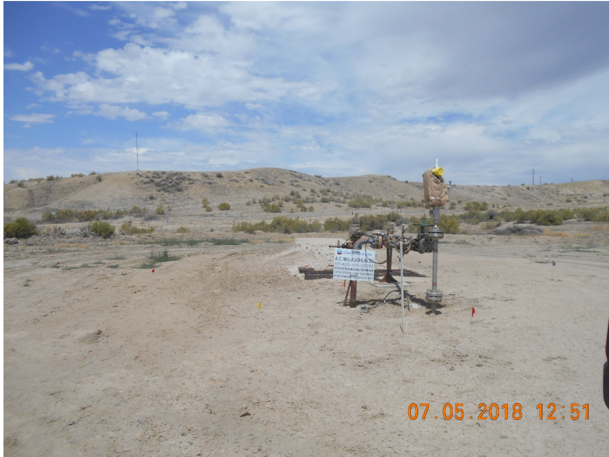
Injection Wellhead
