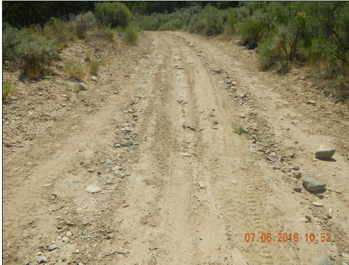
Erosion of ruts on road to location.
