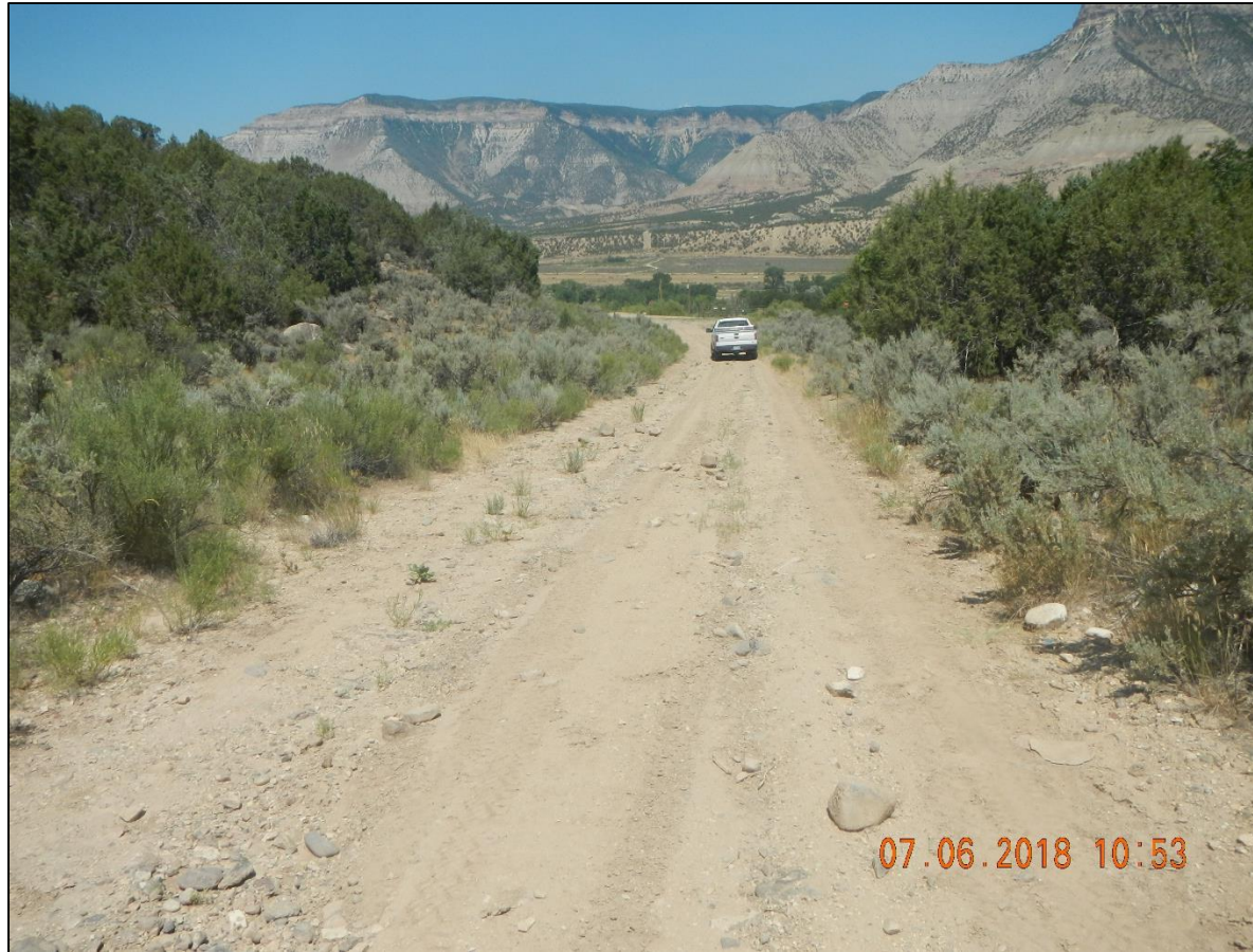
Erosion of ruts on road to location.
