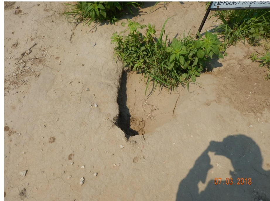
Photo 2: Photo taken at well head. Photo shows subsidence at well.
