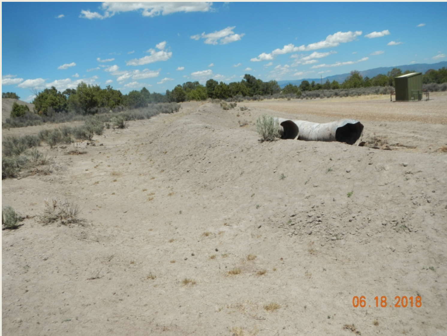
Photo 2. View of berms and diversion in the western project area from the southwestern corner facing northward. Culverts need to be removed.
