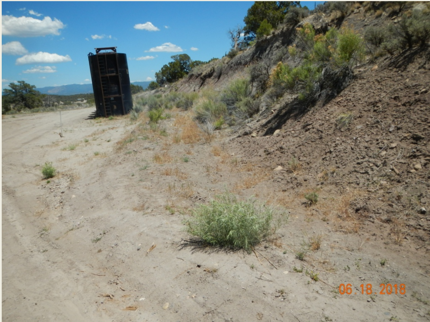
Photo 1. View of the project area from the southwestern corner facing eastward. Southern cut-slope does not appear stabilized as a result of undercutting at the top of the slope and sediment deposition at the toe of the slope. Stormwater controls need to be installed to stabilize erosion on the southern cut-slope
