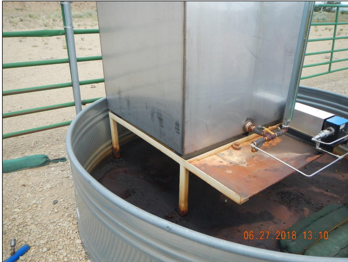
Chemical spill and staining in metal secondary containment.
