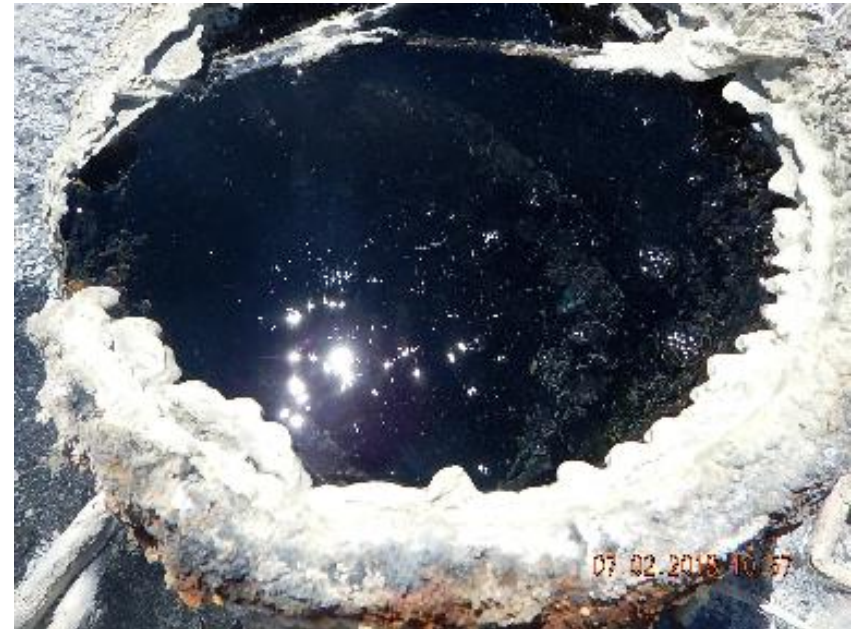
Photo 6: Mineral around lip of casing.
