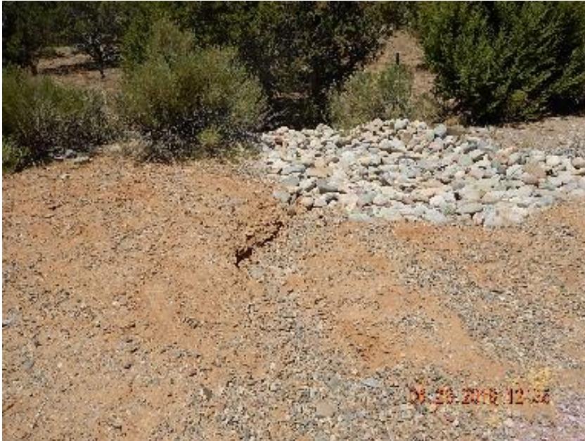
Photo 5: Erosion channel developing at front of rock run down.
