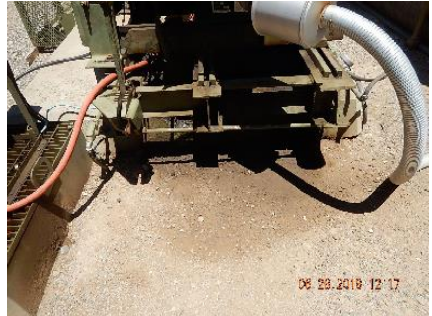
Photo 2: Impacted soil and gravel at rear of pump jack.
