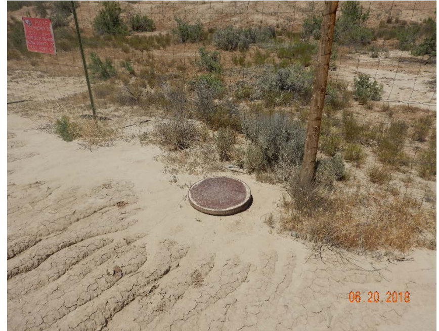
Photo #10 – Evidence of erosion and sediment transport at leak detection system cover on north side of pit
