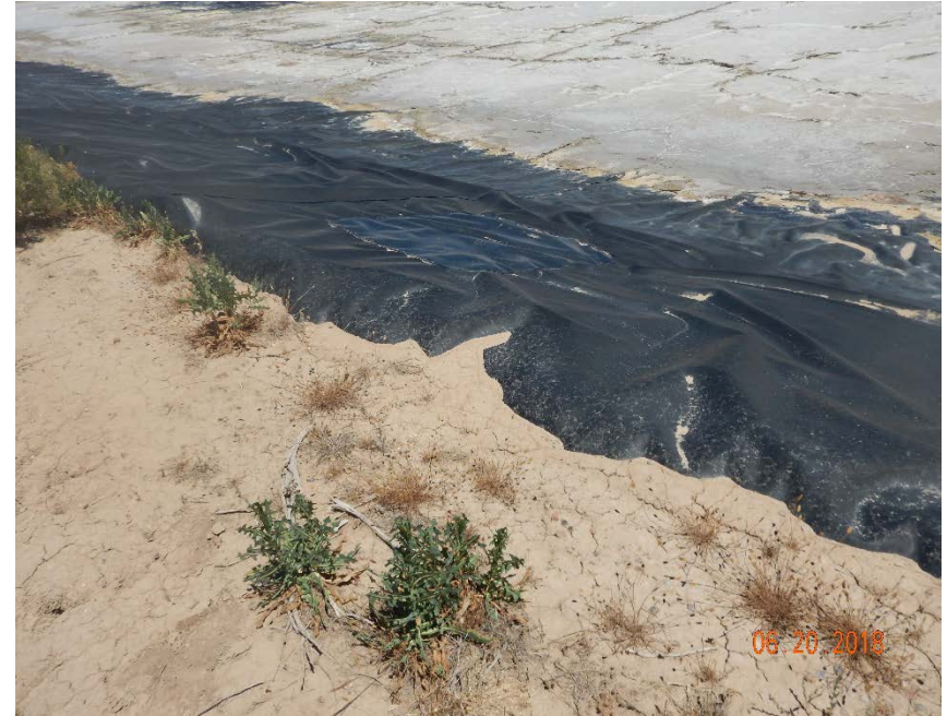
Photo #6 – Weeds and sediment transport encroaching on pit liner (west berm).
