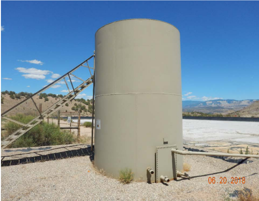
Photo #13 – 300 bbl produced water AST in lined earthen berm at SW corner of pit.
