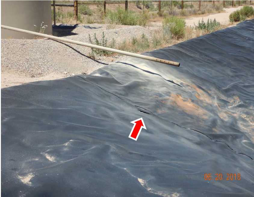
Photo #5 – Torn liner at SW corner of pit, below inlet from produced water tank.
