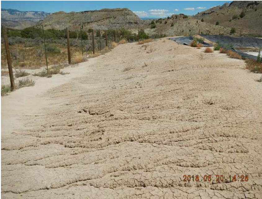
Photo #11 – More berm erosion and off-site sediment transport along north berm.
