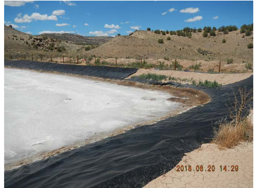
Photo #12 – Weeds growing in compromised liner area at NE corner of pit.
