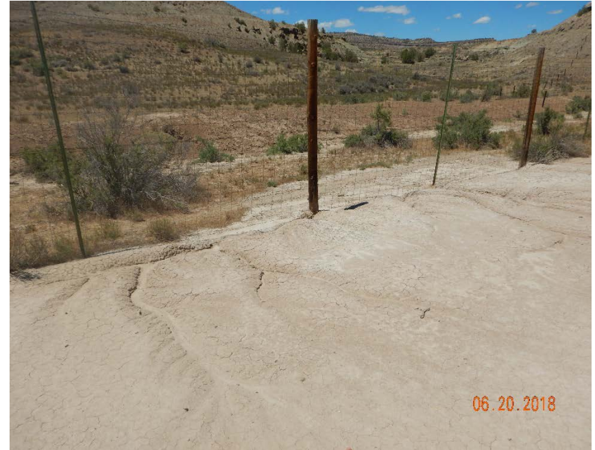
Photo #8 – Berm erosion with off-site sediment transport around pit perimeter (west berm).
