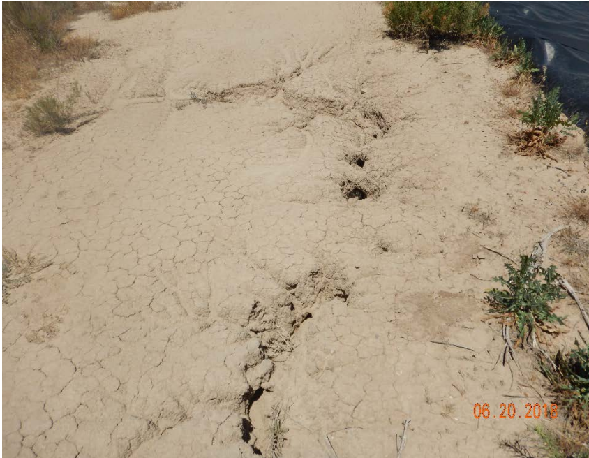
Photo #7 – Erosion on top of west berm.
