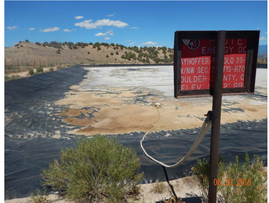
Photo #4 – View from SW corner of pit, looking north. Note sediment and salt remain on top of pit liner and weeds are encroaching along pit perimeter.
