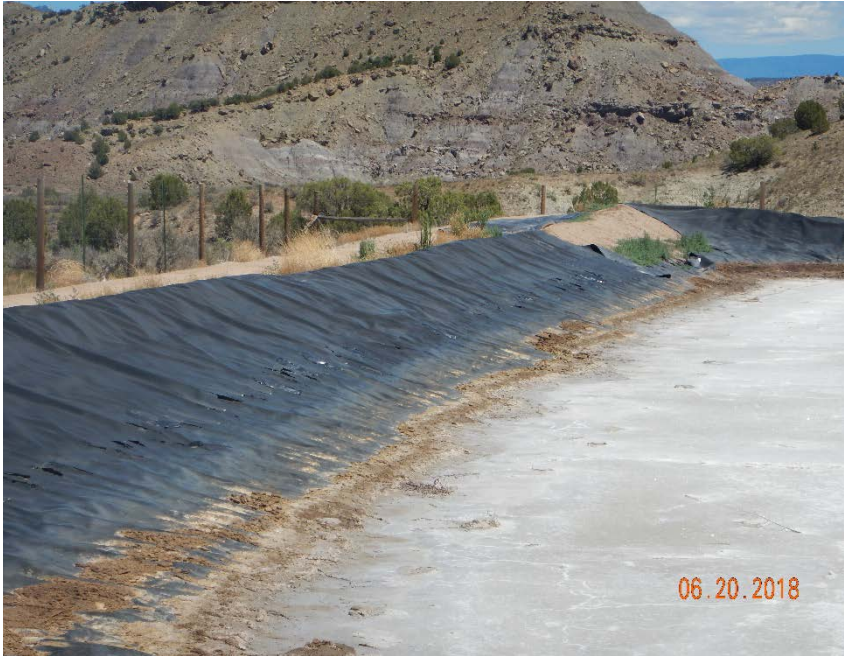
Photo #9 – Pit liner remains compromised at NE corner, as first indicated in December 19, 2017 Field Inspection Report #689100109.
