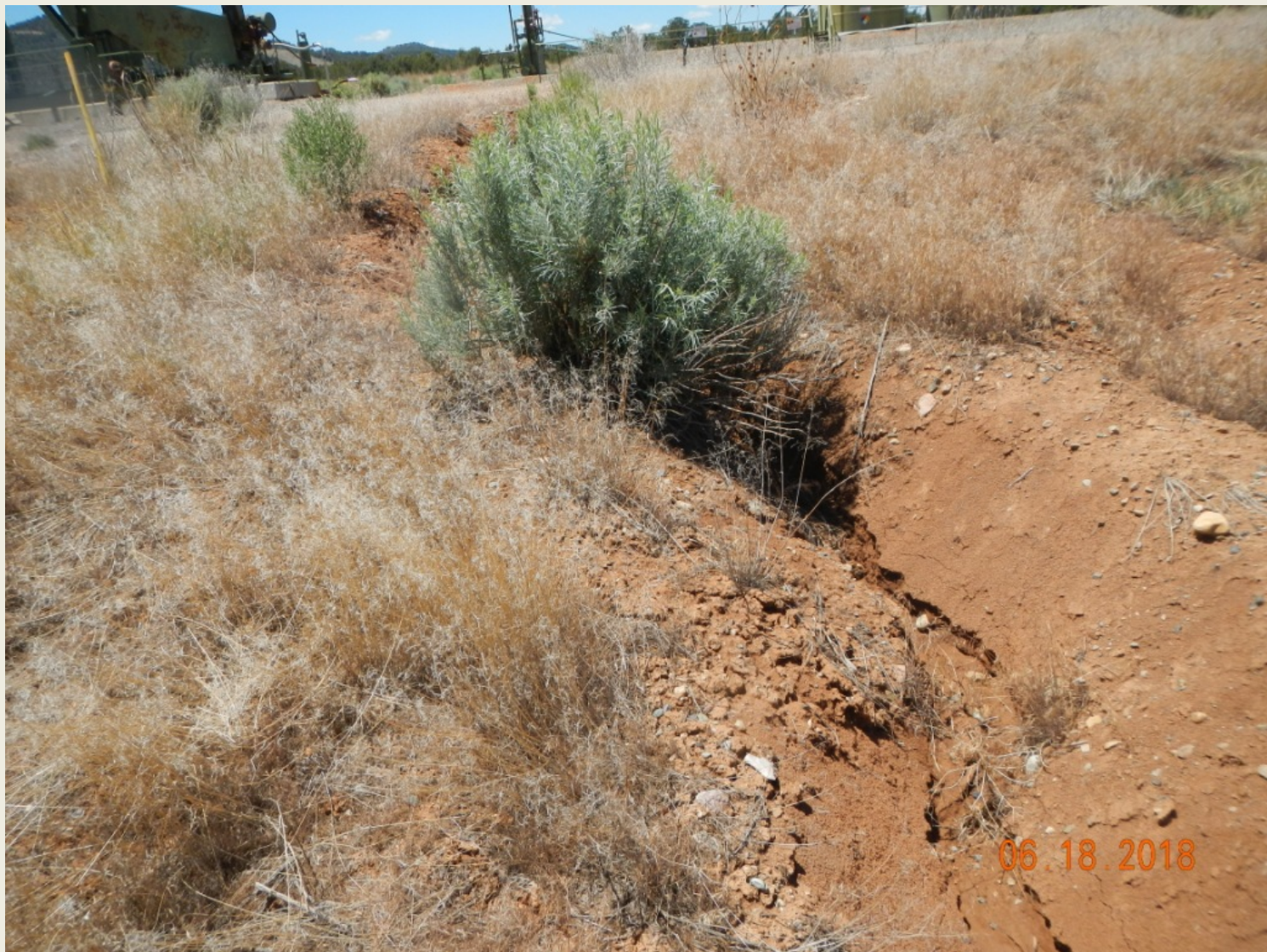
Photo 5. View erosional channel approximately 2.5 feet wide and deep in the northern portion of the project area. Stormwater controls are needed to stabilize erosion here.
