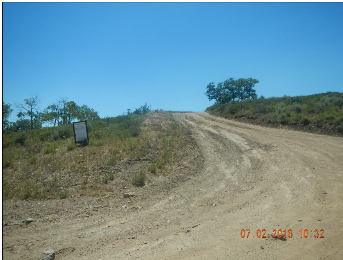
Deep ruts at access and main road intersection.
